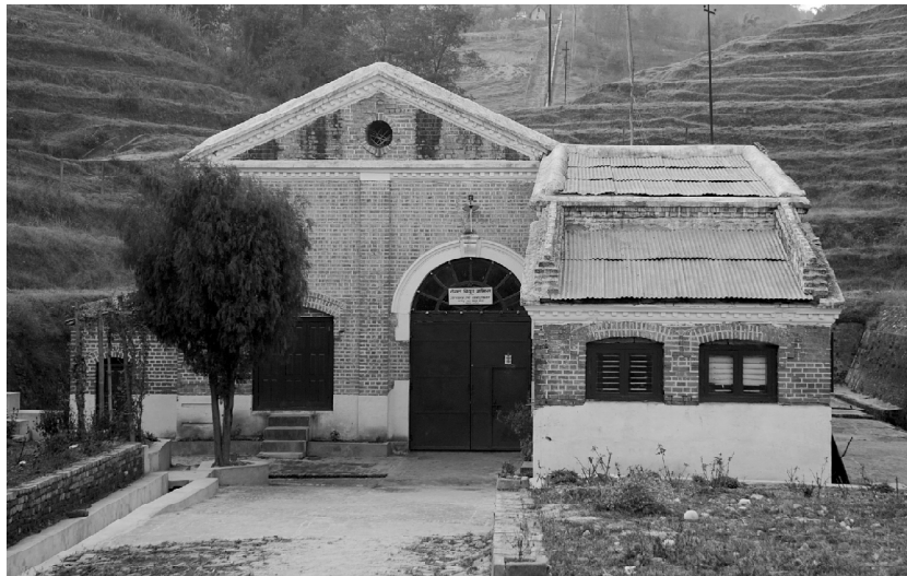
Pharping Hydro-electric Power House
