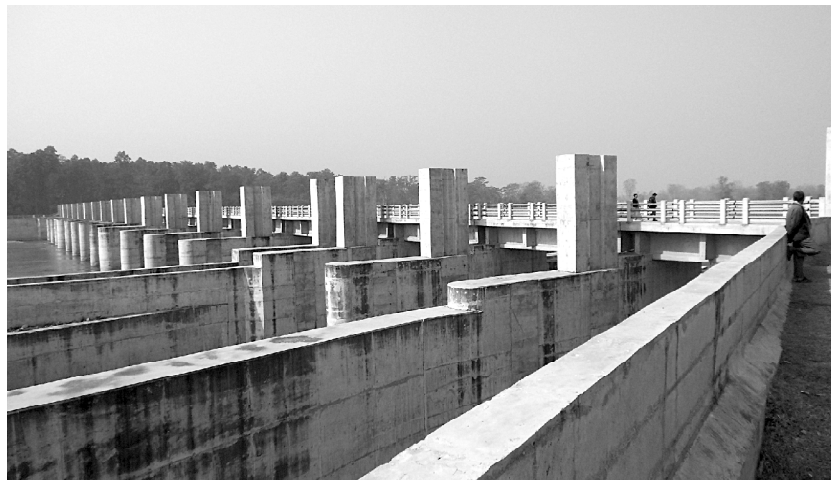
Sikta Irrigation Project
