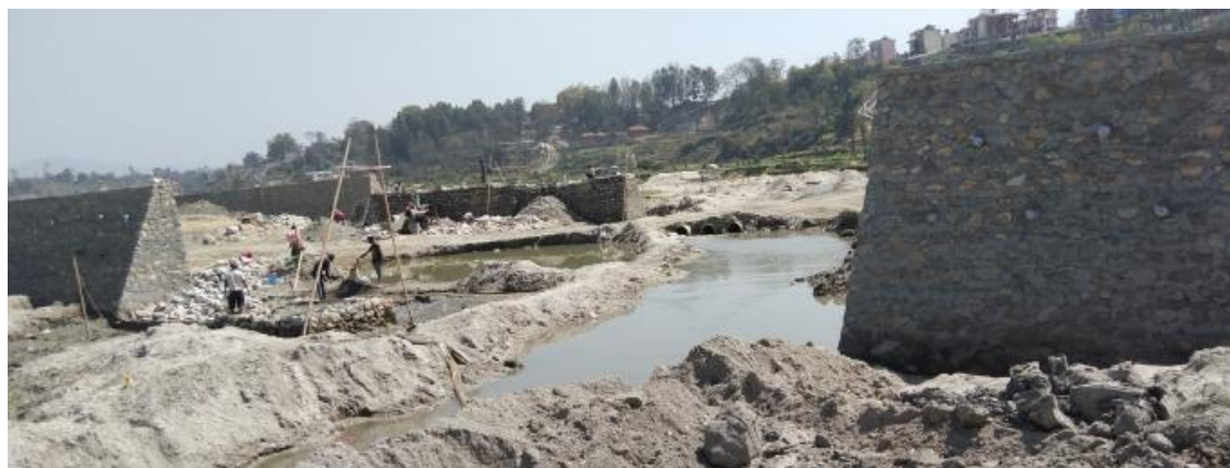
Figure 3-18: River training works in Manohara
