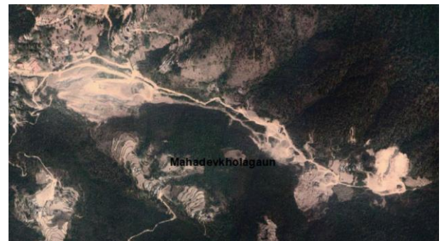
Figure 5-12: Hillslope excavation in Nakhu upstream
