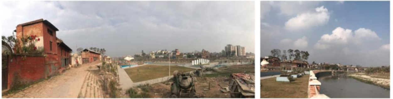
Figure 3-20: Left: Shankha Park constructed on the reclaimed land, also seen are stone steps and bhakaro with few old house along the edge: Right: The width of the river is controlled using vertical walls and seen are the parapet walls along the Sankha Park.
