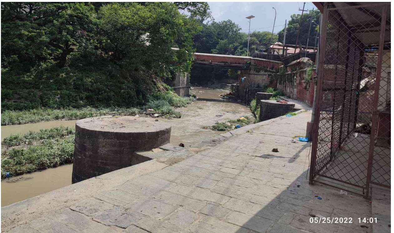
Narrow section at d/s Bagmati Khola at Gaurighat area
