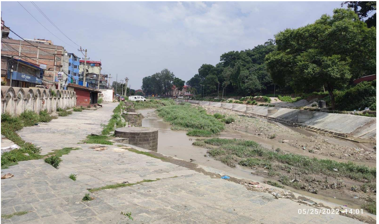
Wide section at u/s of Bagmati Khola near Gaurighat
