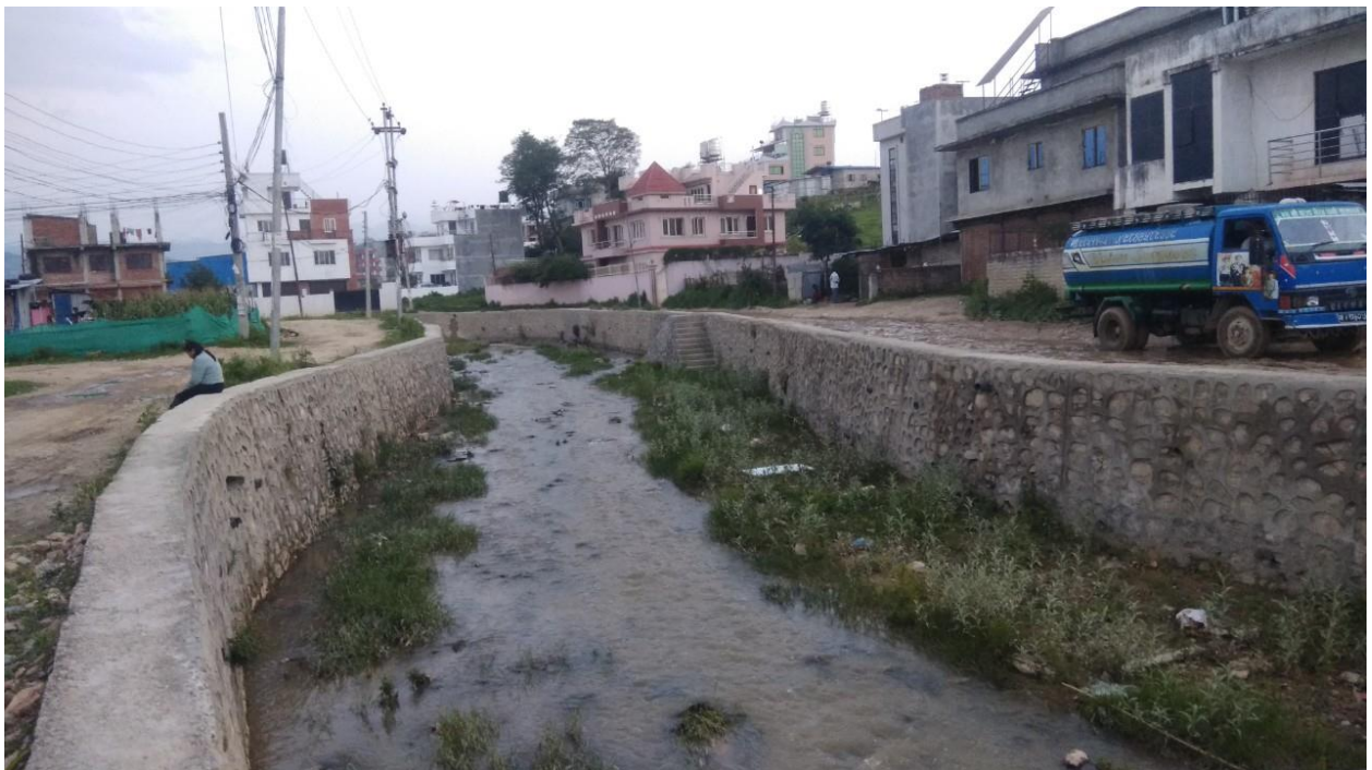
River Training Works- Stone Masonry Wall in Kodku Khola (Karmanasa)
