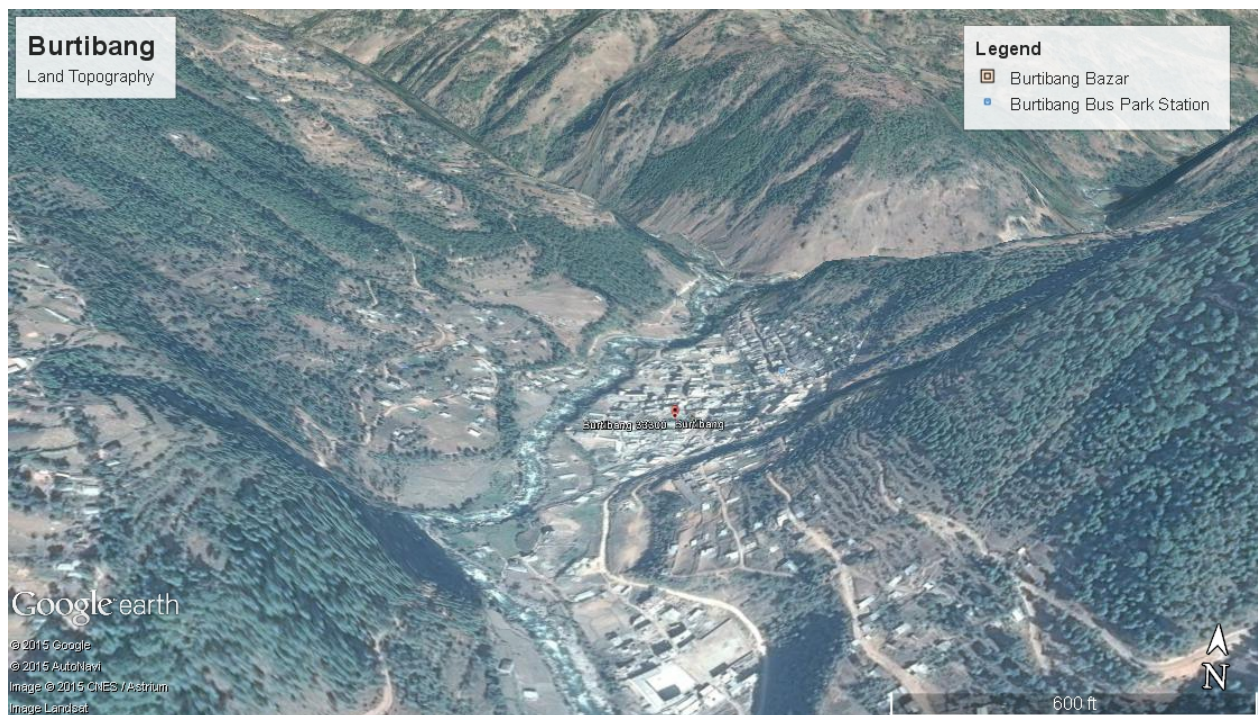
Figure 15 Land Topography of Burtibang, Baglung( Source: Google Earth)
