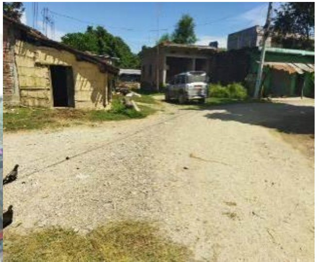
Structure at RoW on Tilottama-10
