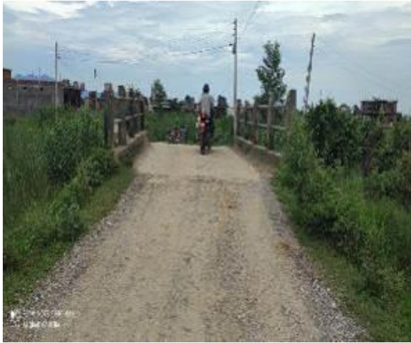
Bridge Structure at RoW
