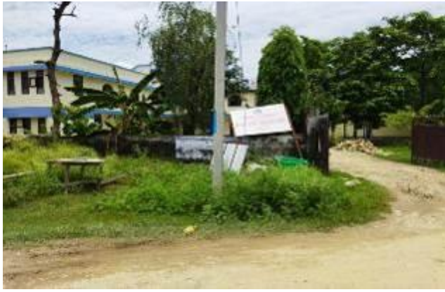
Pole at RoW
