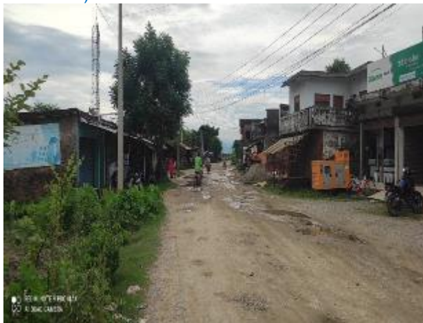
- Tree within the RoW to be removed
