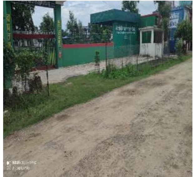
Condition of existing road
