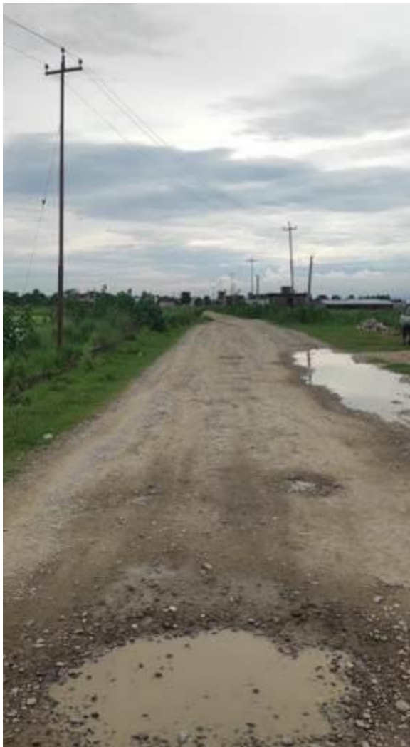
Condition of existing road
