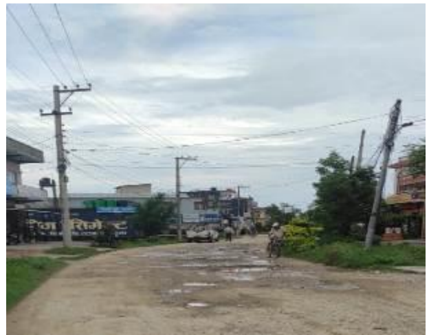
- Existing condition of the road
