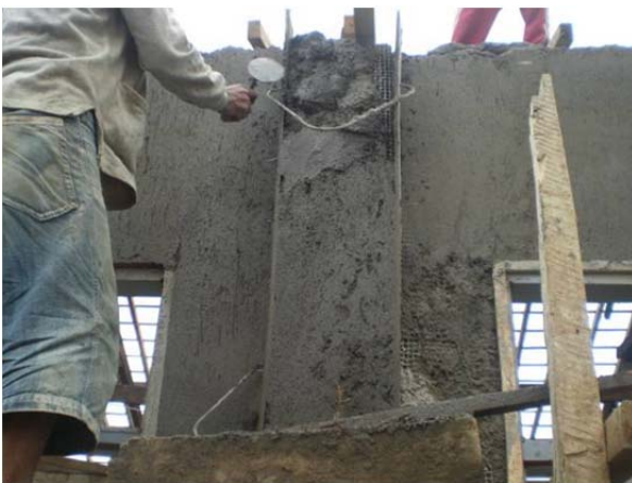
Figure B-9: Retrofitting works for the wall
