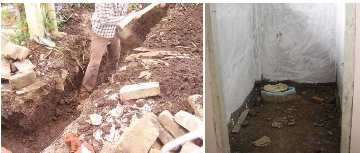
Figure B-11: Sanitary works (drainage system (left) and toilet (right))
