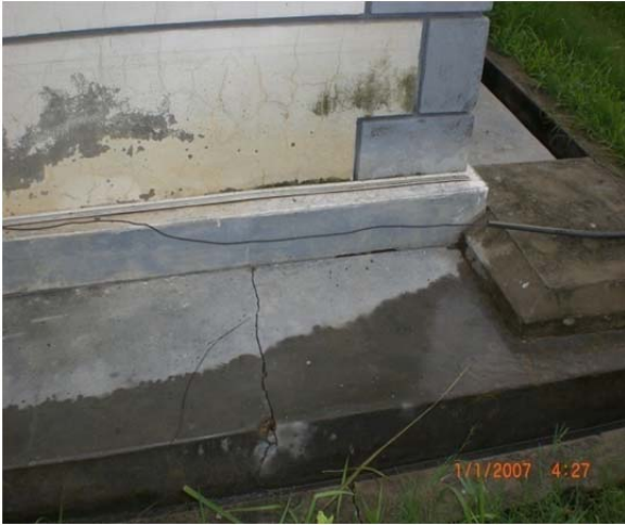
Figure B-21: Crack at Plinth Protection.
