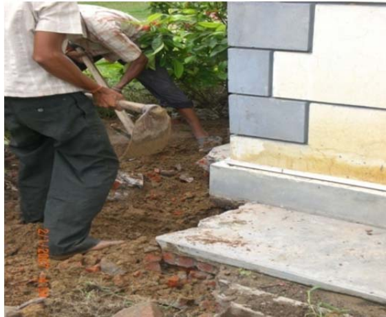
Figure B-16: Excavation for Foundation depth check
