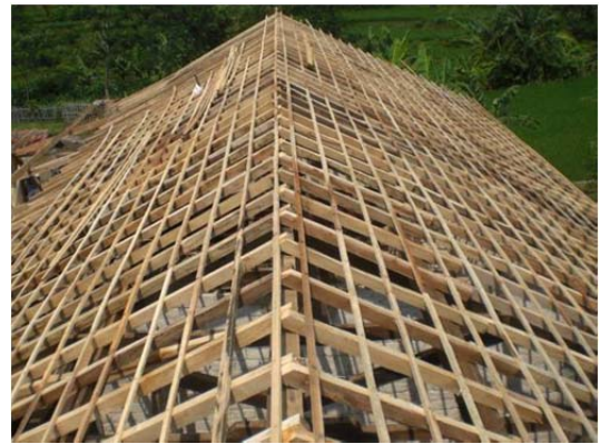
Figure B-12: Retrofitting works for the trusses and roof (providing proper materials and detailing)
