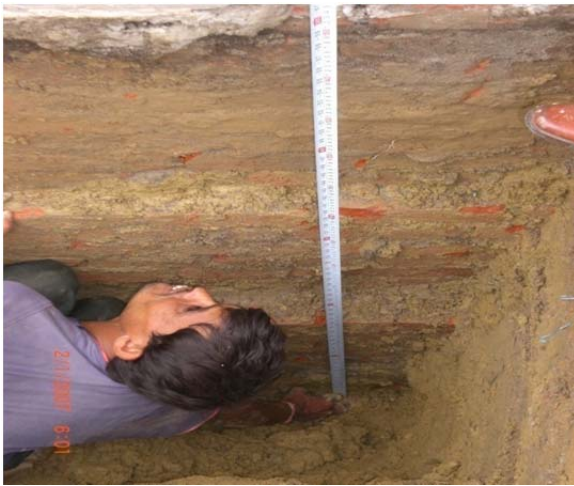
Figure B-17: Foundation Exploration
