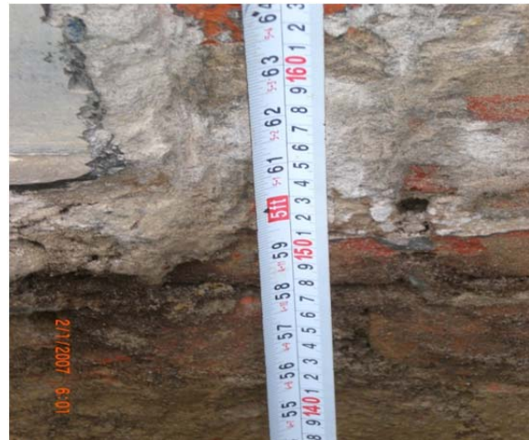
Figure B-18: Tie Beam Exploration
