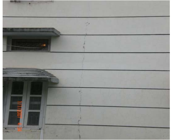
Figure B-22: Vertical crack on wall due to pipe duck
