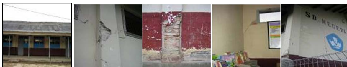
Figure B- 3: Existing Condition of SDN Padasuka II
