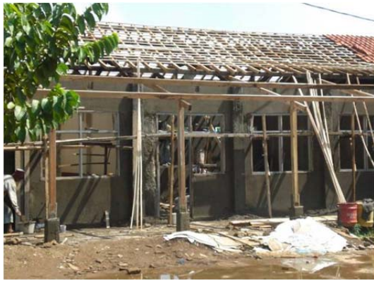
Figure B-12: Retrofitting works for the trusses and roof (providing proper materials and detailing)
