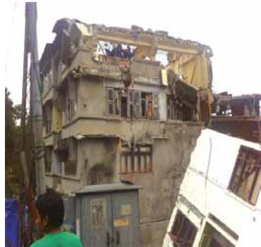
Figure 5.4 Damage grade 4 (source: MRB & Associates)
