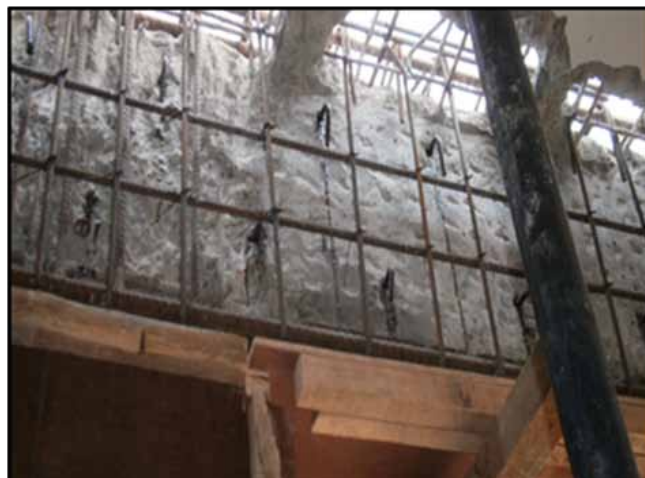
Figure 2.1 Anchors driven inside concrete after placing epoxy resin
