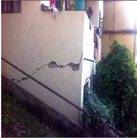
Figure 5.3 Damage grade 3 (source: MRB & Associates)
