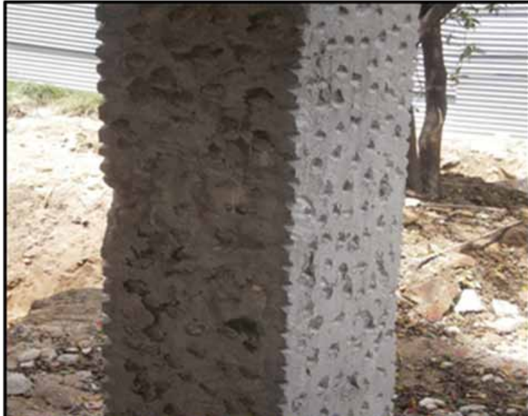
Figure 2.2 Roughing of concrete surface for proper bondage with new concrete
