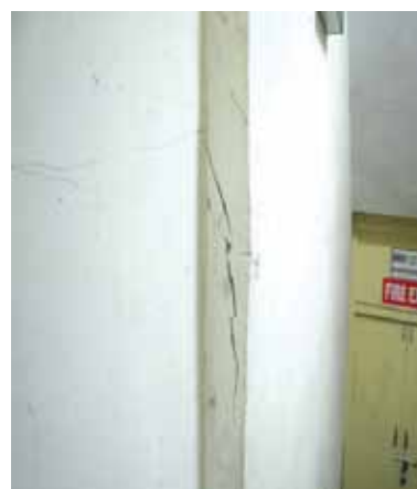
Figure 5.2 Damage grade 2 (source: MRB & Associates)
