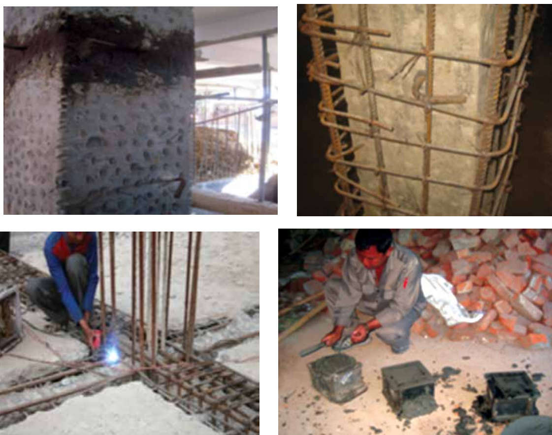
Figure 6.6 Strengthening of original structure (Source: MRB & Associates)
