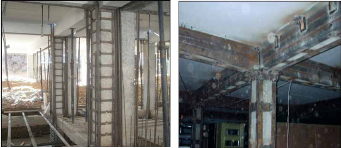
Figure 6.10 Steel jacking of columns (source: MRB & Associates)
