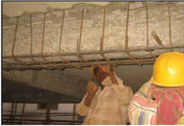
Figure 6.12 Reinforcement placing for beam jacketing (source MRB & Associates)
