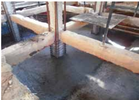
Foundation retrofit with concrete
