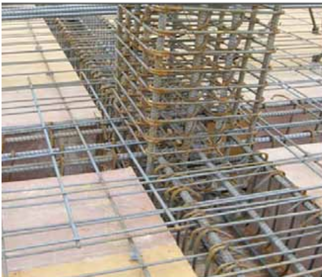
Figure 6.32 Beam column joint detailing (source: MRB & Associates)
