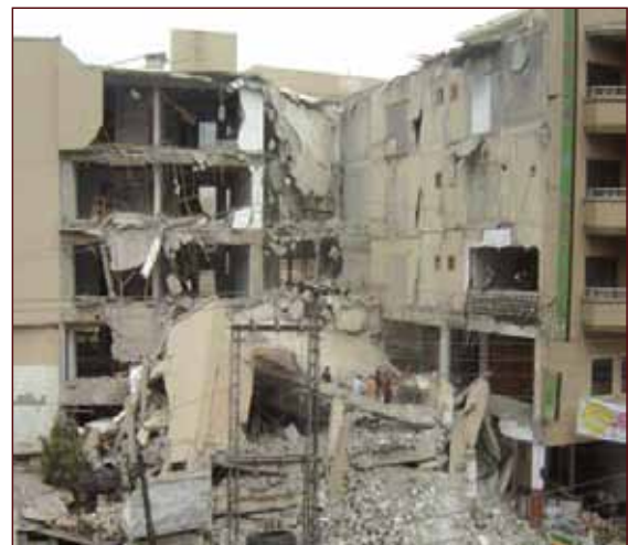
Figure 5.5 Damage grade 5 (source: MRB & Associates)
