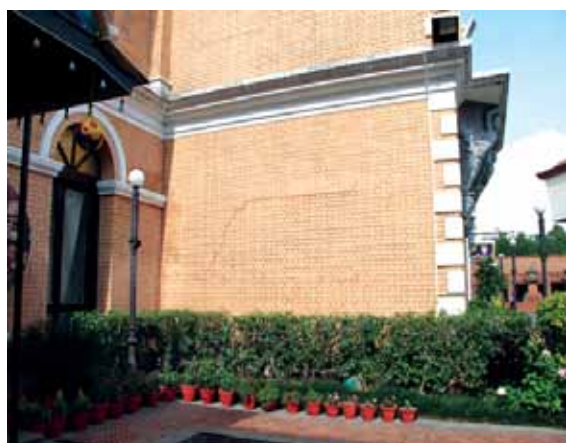
Figure 5.2 Damage grade 2 (source: MRB & Associates)
