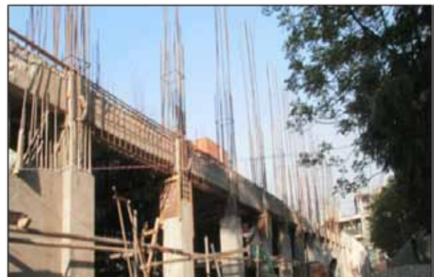
Figure 6.15 Encasement of existing beam (Source: MRB & Associates)
