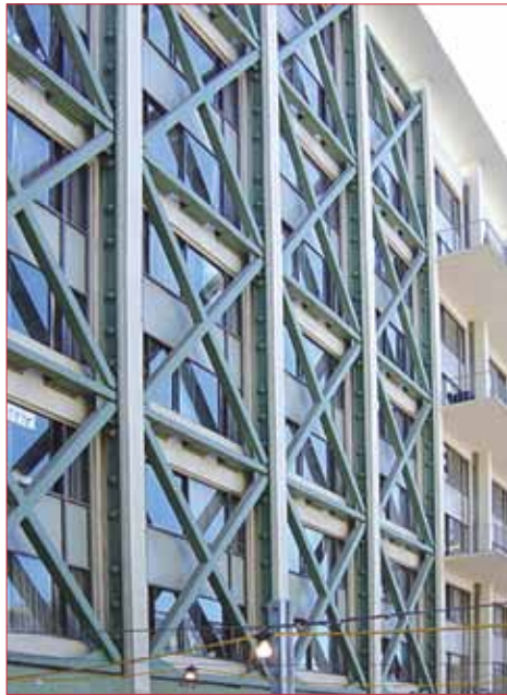
Figure 6.31 Addition of steel bracing
