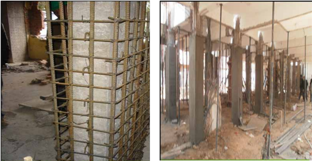
Figure 6.8 Jacketing of column (source MRB & Associates)
