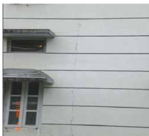
Figure 5.1 Damage grade 1 (source: MRB & Associates)
