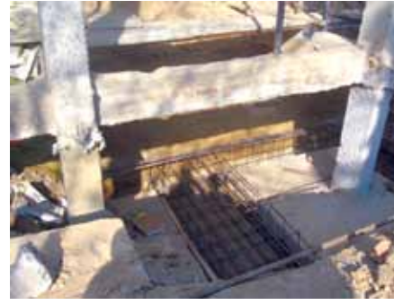
Reinforcement layout at foundation for retrofit
