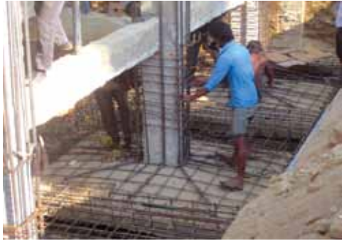
Reinforcement layout at foundation for retrofit
