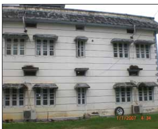
Figure 5.1 Damage grade 1 (source: MRB & Associates)
