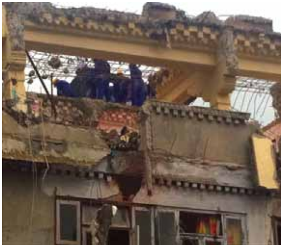
Figure 5.4 Damage grade 4 (source: MRB & Associates)
