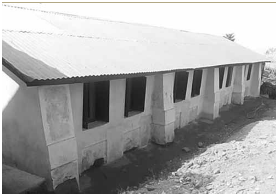
Figure 6.2 Buttress provide to exterior building (source: Hari Darshan Shrestha)
