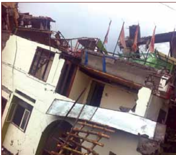
Figure 5.5 Damage grade 5 (source: MRB & Associates)
