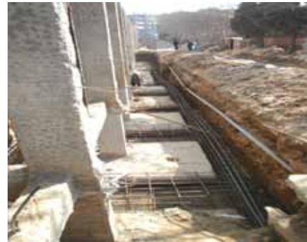
Reinforcement layout at foundation for retrofit
