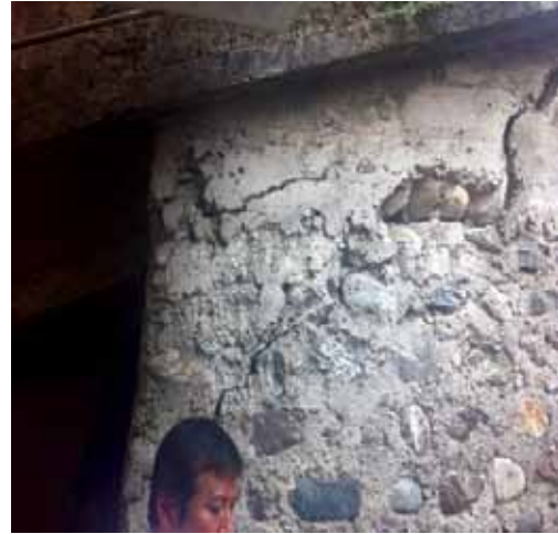
Figure 5.3 Damage grade 3 (source: MRB & Associates)
