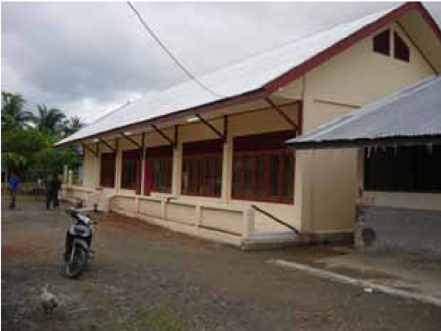
Figure A-43 Retrofitted Structure
