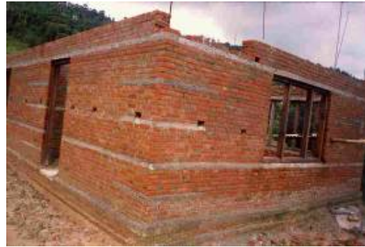
Fig 2.16 (b) Presence of Sill Band, Corner Stitch and Lintel Band
