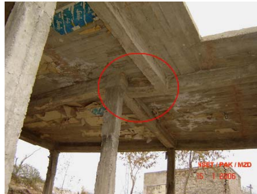
Fig 2.1 (b) Beam Resting on Beam
