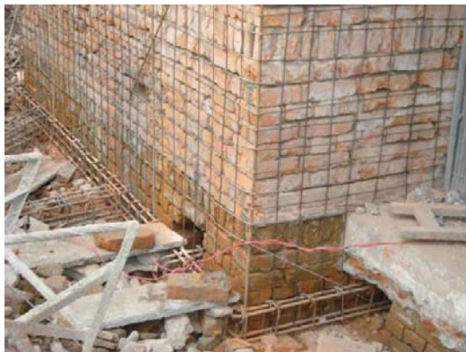
Fig 5. (b) Erection of Reinforcement for Wall Jacketing
