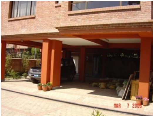
Fig 2.5 (c) Soft Storey Problem due to Lack of Brick Infill in Ground Floor
