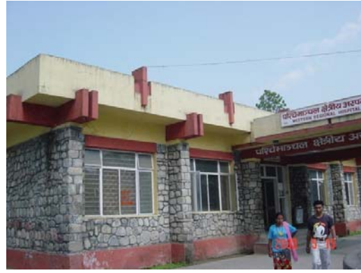
Fig 1.2 (b) Stone in Cement Building
