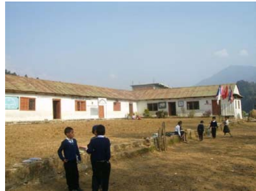
Fig 2.3 (b) L-Shaped School Building Irregularities in Shape
