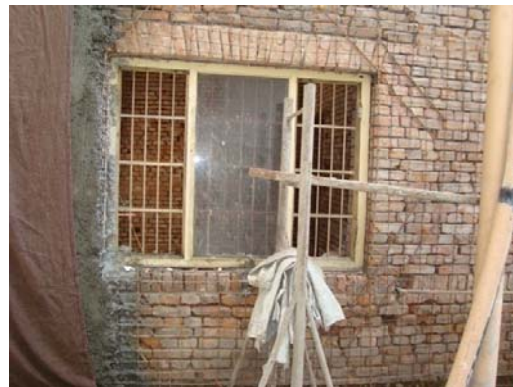
Fig 5. (c) Wall Jacketing in Process
