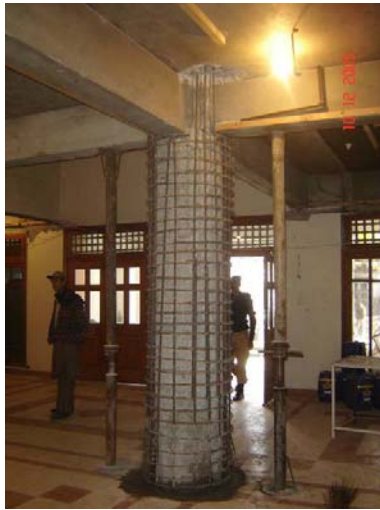
Fig 10. (a) Jacketing of RC Column
