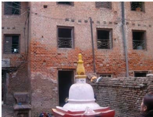
Fig 2.10 Problem due to Deterioration of Masonry Units and Joints
