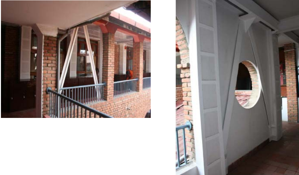
Fig. 11. Retrofitting by Diagonal Steel Bracing
