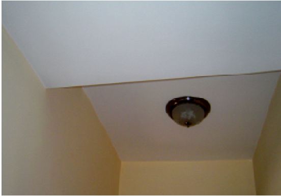
Fig 2.17 (a) Drop in Floor Slab
