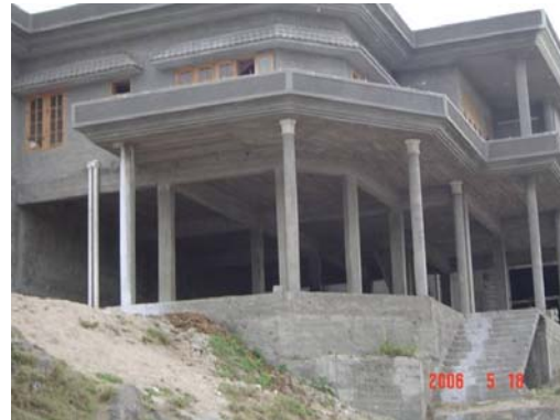
Fig 2.5 (c) Soft Storey Problem due to Lack of Brick Infill in Ground Floor
