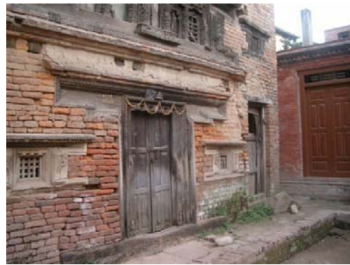
Fig 2.10 Problem due to Deterioration of Masonry Units and Joints
