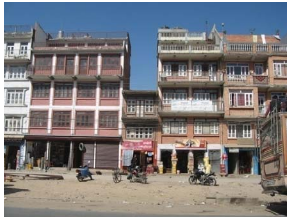
Fig 2.2 (e) Buildings Attached to Each Other Without Seismic Gap (These buildings are liable to suffer in pounding)
