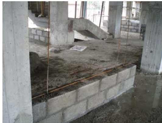
Fig 2.12 (b) Tying of Infill Wall with Frame
