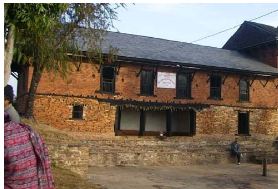
Fig 1.5 (a) Stone in Mud in Ground Floor and Brick in Mud in First Floor
