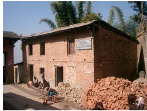
Fig 1.1 (b) Brick in Mud Building
