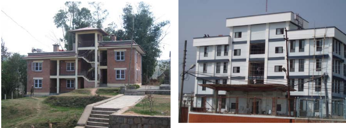
Fig 1.4 Engineered Reinforced Concrete Moment Resisting Frame Buildings
