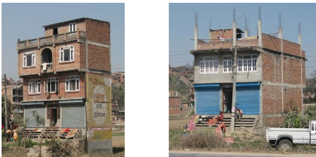
Fig 1.3 Non Engineered Reinforced Concrete Moment Resisting Frame Buildings
