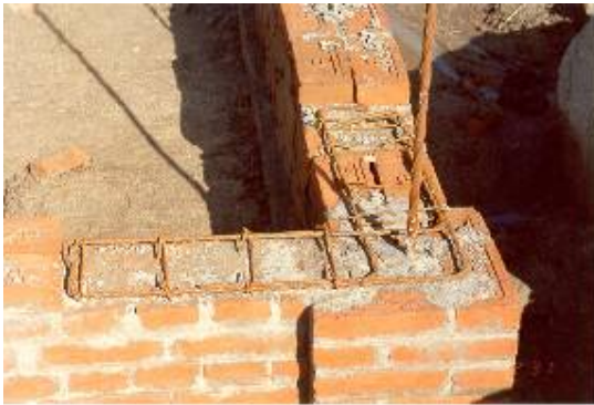
Fig 2.16 (a) Vertical Reinforcement and Corner Stitch
