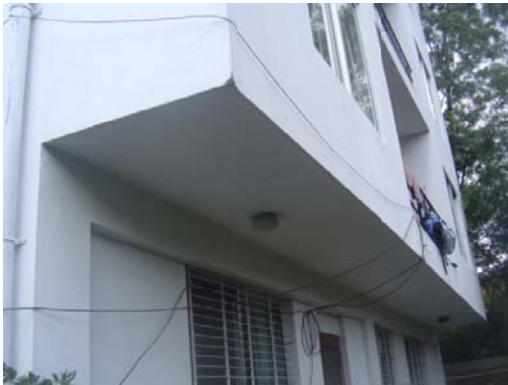
Fig 2.1 (a) Full Brick Wall on Cantilever Slab Projection
