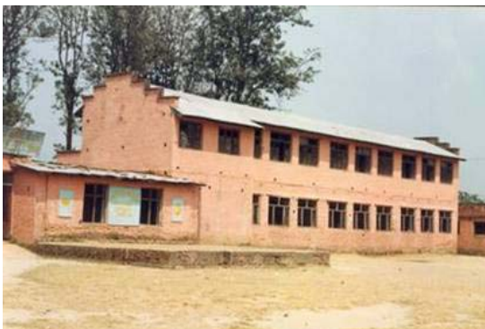
Fig 2.15 (a) Large Window Openings in Masonry Walls
