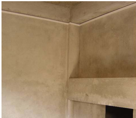
Fig 2.13 (a) Beam at Mid Height of Column
