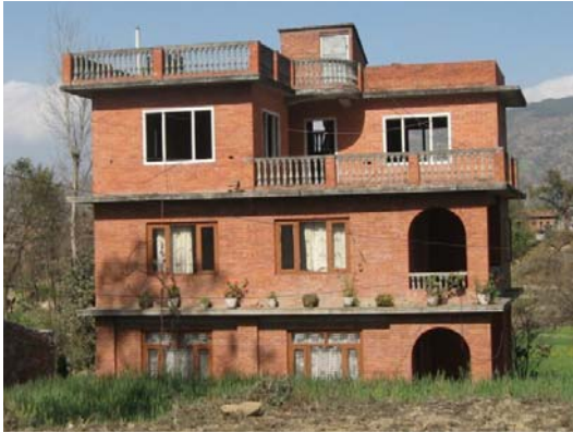
Fig 1.2 (a) Brick in Cement Building
