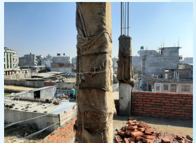
Figure 17: - Curing in column and slab
