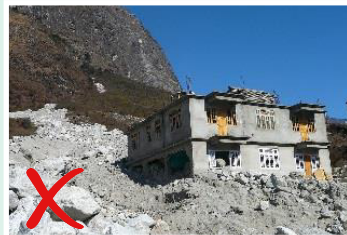
rock fall area
