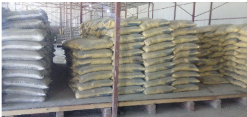
Figure 4: - Systematic storage of cement bags at a construction site
