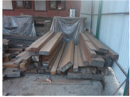
Figure 13: - Proper storage of timber
