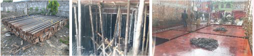
Figure 11: - Steel poles and planks used as scaffolding and formwork
