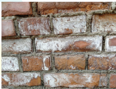
Figure 6: - White powder (Efflorescence) seen on wall and brick
