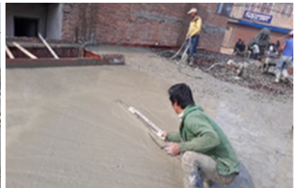
Figure 15: - Compaction and levelling after pouring concrete
