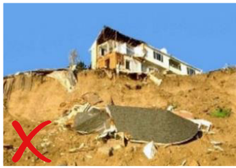
Landslide prone area
