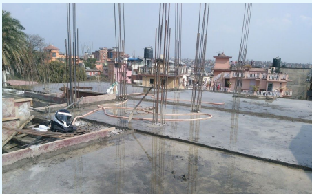
Figure 17: - Curing in column and slab
