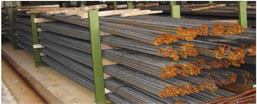
Figure 10: - Storage of reinforcement at a construction site
