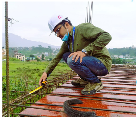
Figure 1: An engineer checking and supervising whether the building is constructed as per the design drawing or not
