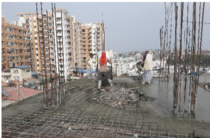
Figure 15: - Compaction and levelling after pouring concrete
