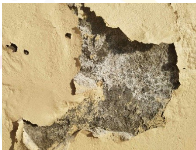
Figure 6: - White powder (Efflorescence) seen on wall and brick
