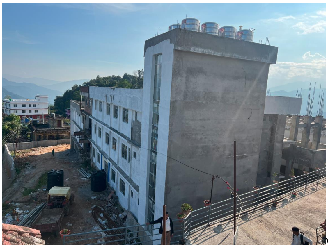
New Building under Construction
