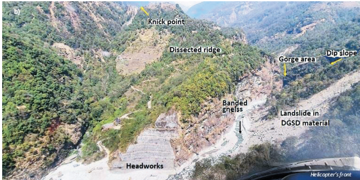
Figure 9: Upstream View of Headworks and Gorge Area
