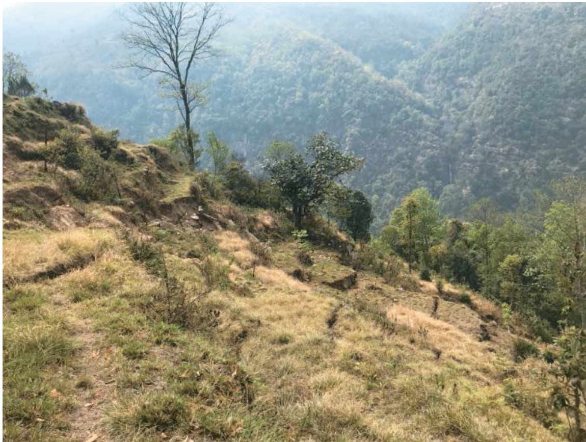
Figure 8.1: Tension Cracks above the Melamchi Left Bank Landslide
