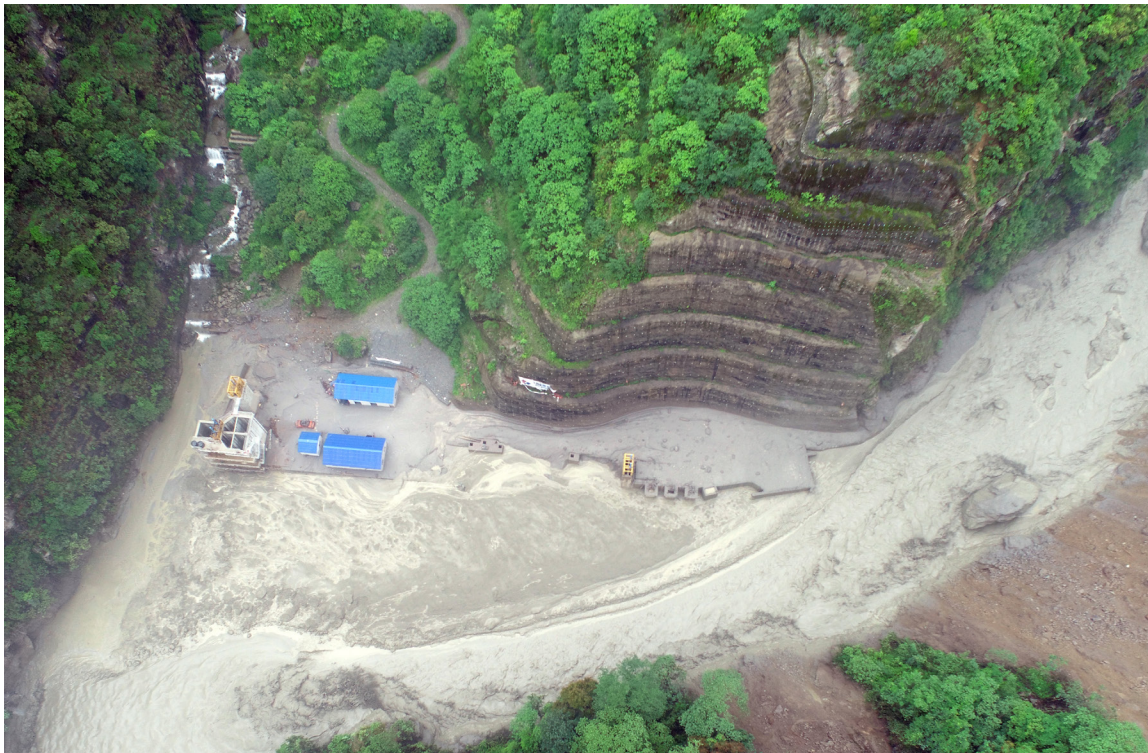
Figure 28: Headworks Shown Partially Buried after June 2021 Flood
