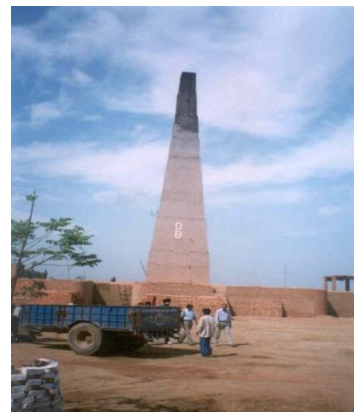
Figure 4.13: Improved Fixed Chimney
