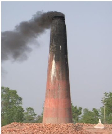
Figure 4.12: Conventional Fixed Chimney
