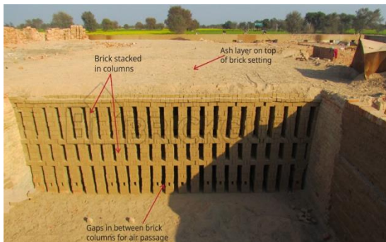
Figure 4.15: Straight Line Brick Setting
