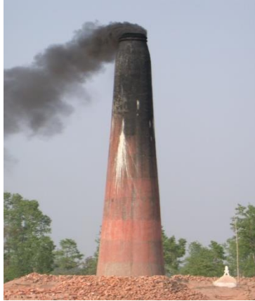
Figure 4.12: Conventional Fixed Chimney
