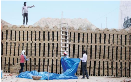
Figure 4.15: Straight Line Brick Setting
