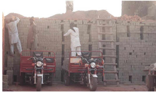
Figure 4.16: Zigzag Brick Setting (Chamber system)
