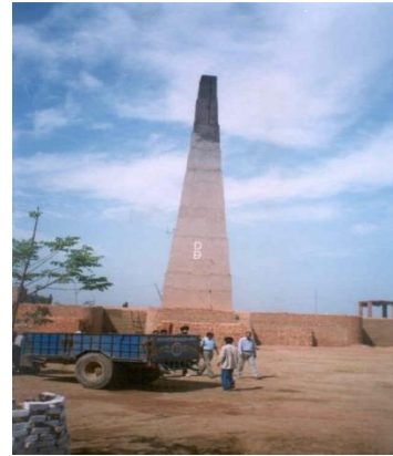
Figure 4.13: Improved Fixed Chimney
