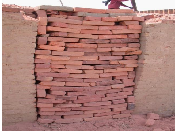
Figure 4.20: Conventional type wicket wall
