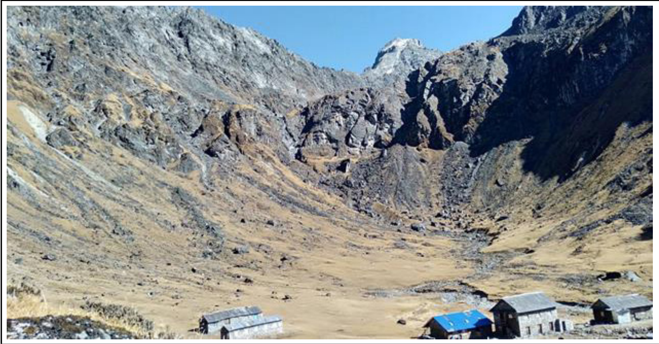
Encroachment at Khola Kharka
