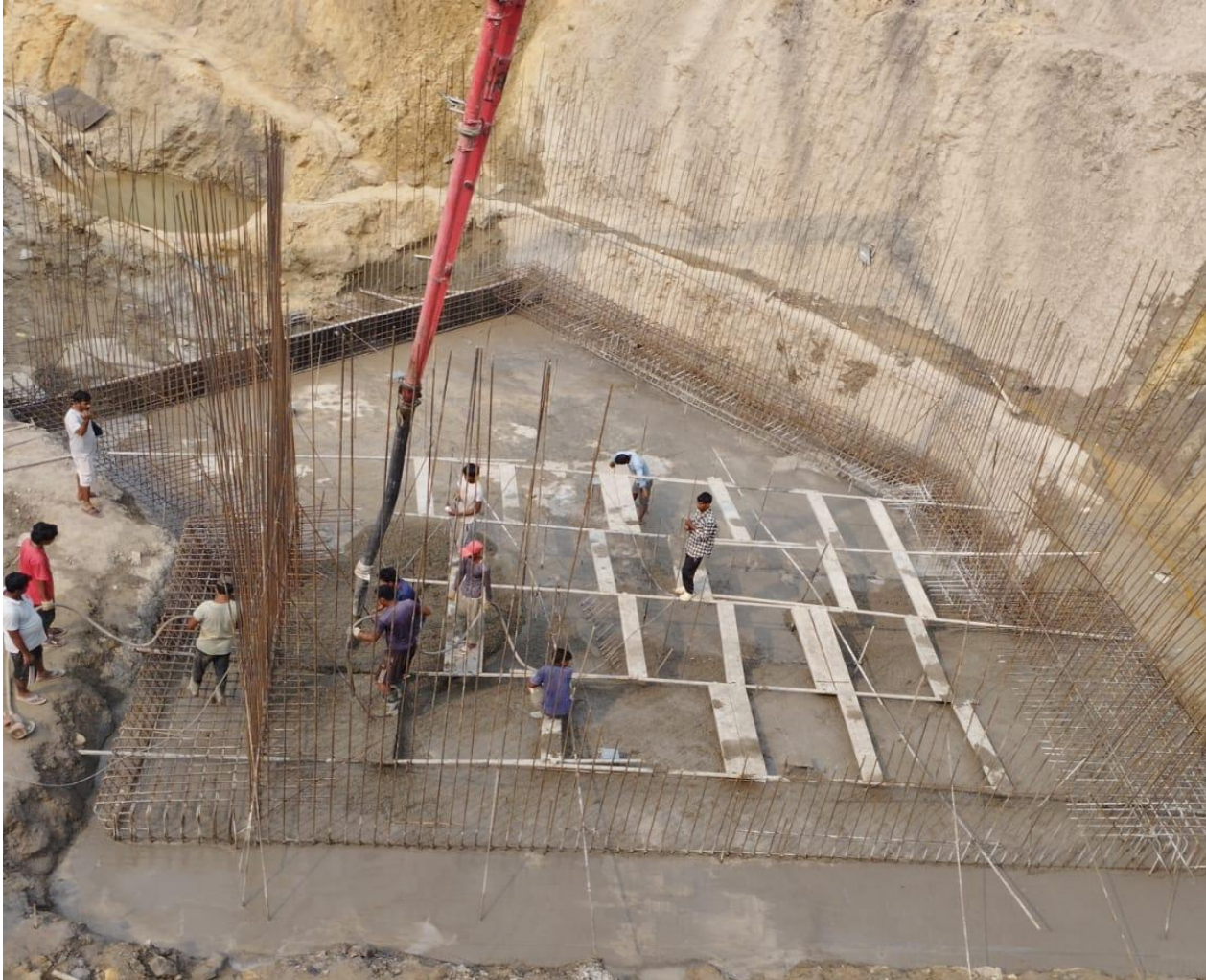
Figure 9 Anchor Block-2 Concreting work recent progress
