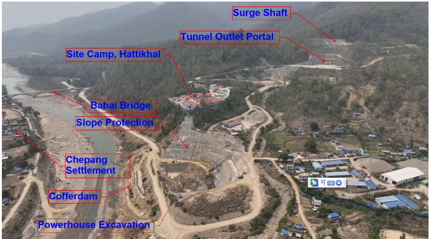
Figure 7 Bird Eye View of Powerhouse, Tunnel inlet and Surge shaft
