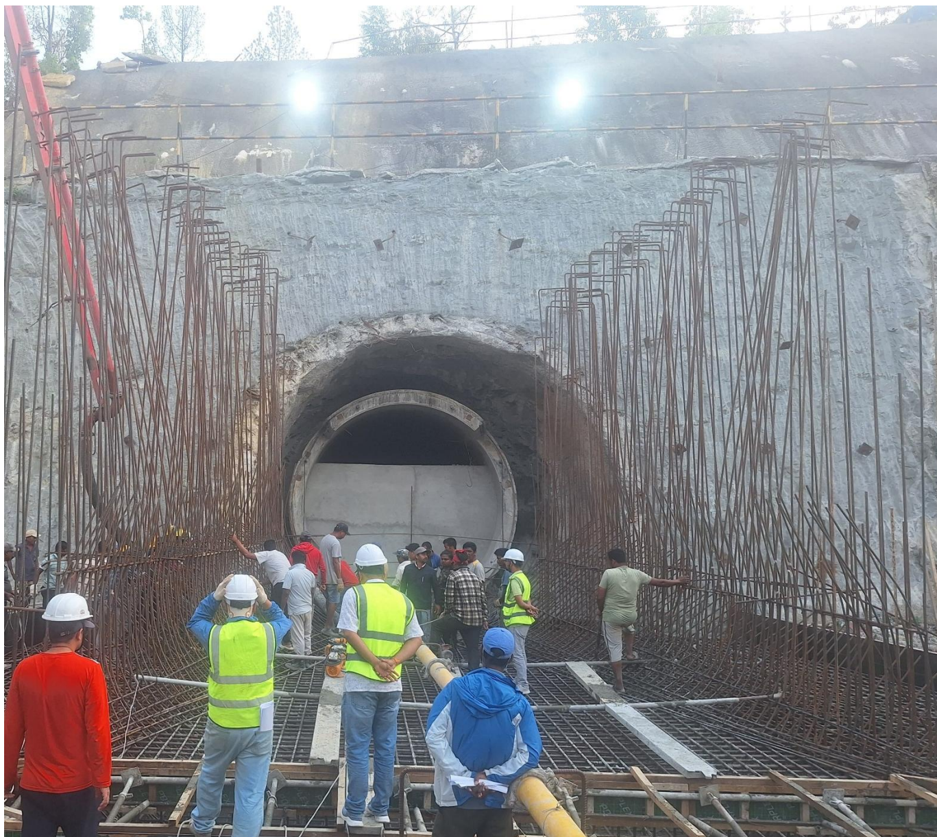
Figure 7 Forebay at Inlet Tunnel Portal
