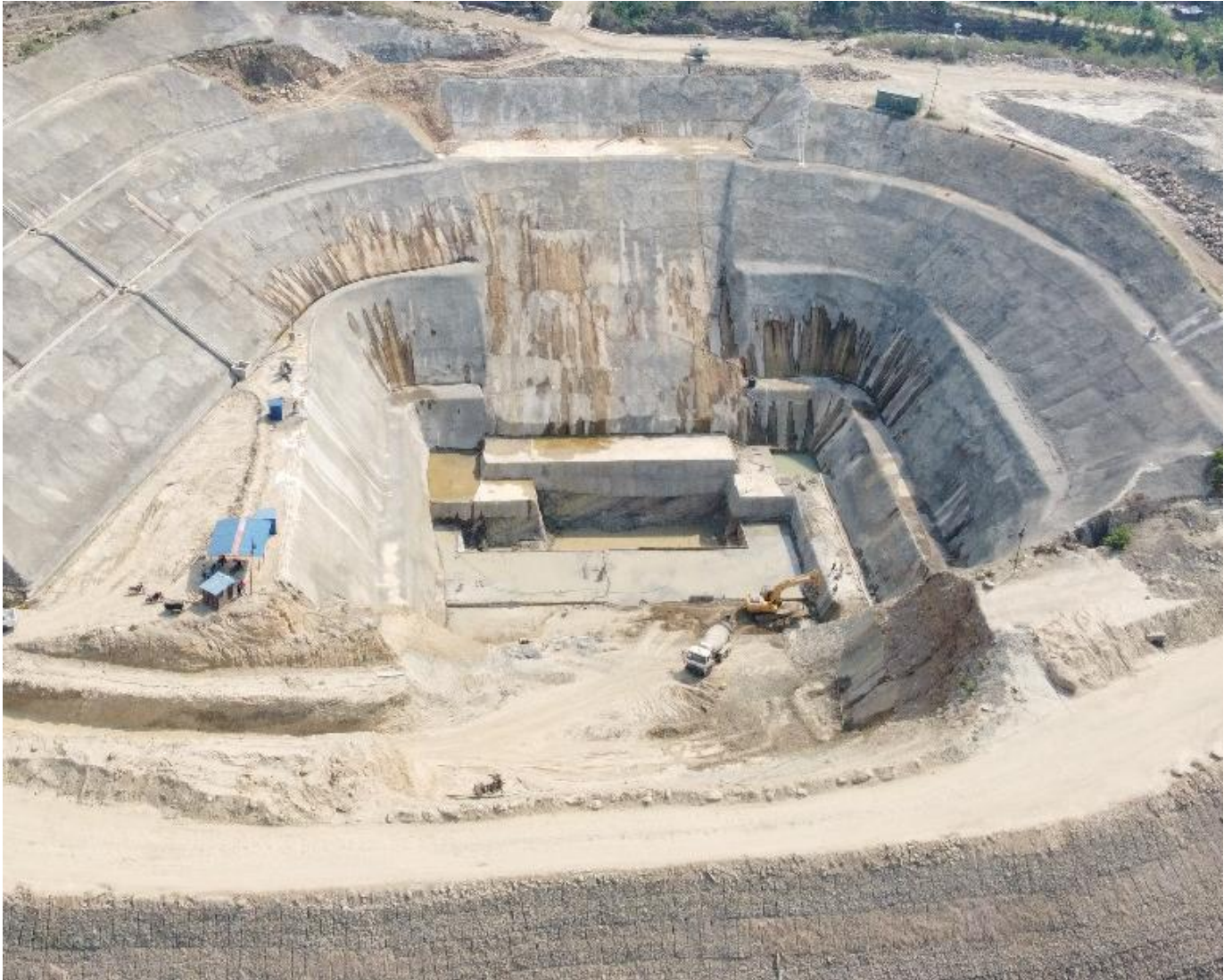
Figure 8 Ongoing Powerhouse Foundation and Slope Protection Works
