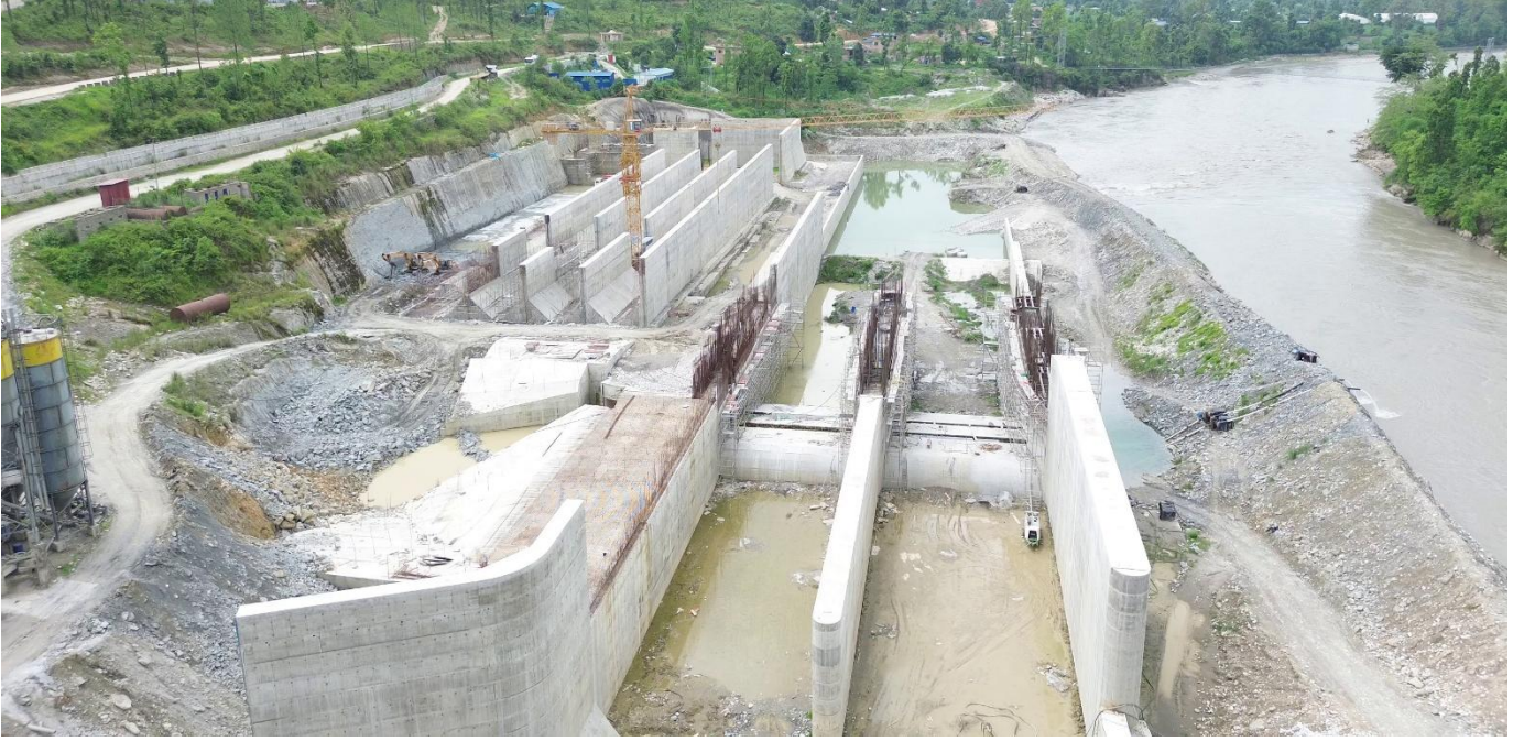
Figure 1 Bird Eye View of Headworks Showing Progress
