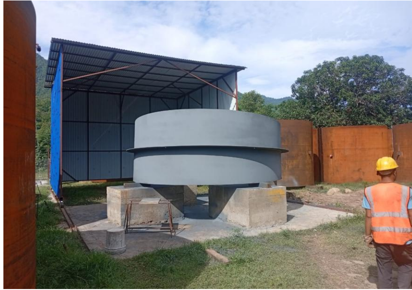
Figure 14 Bending for Penstock Pipe at Site
