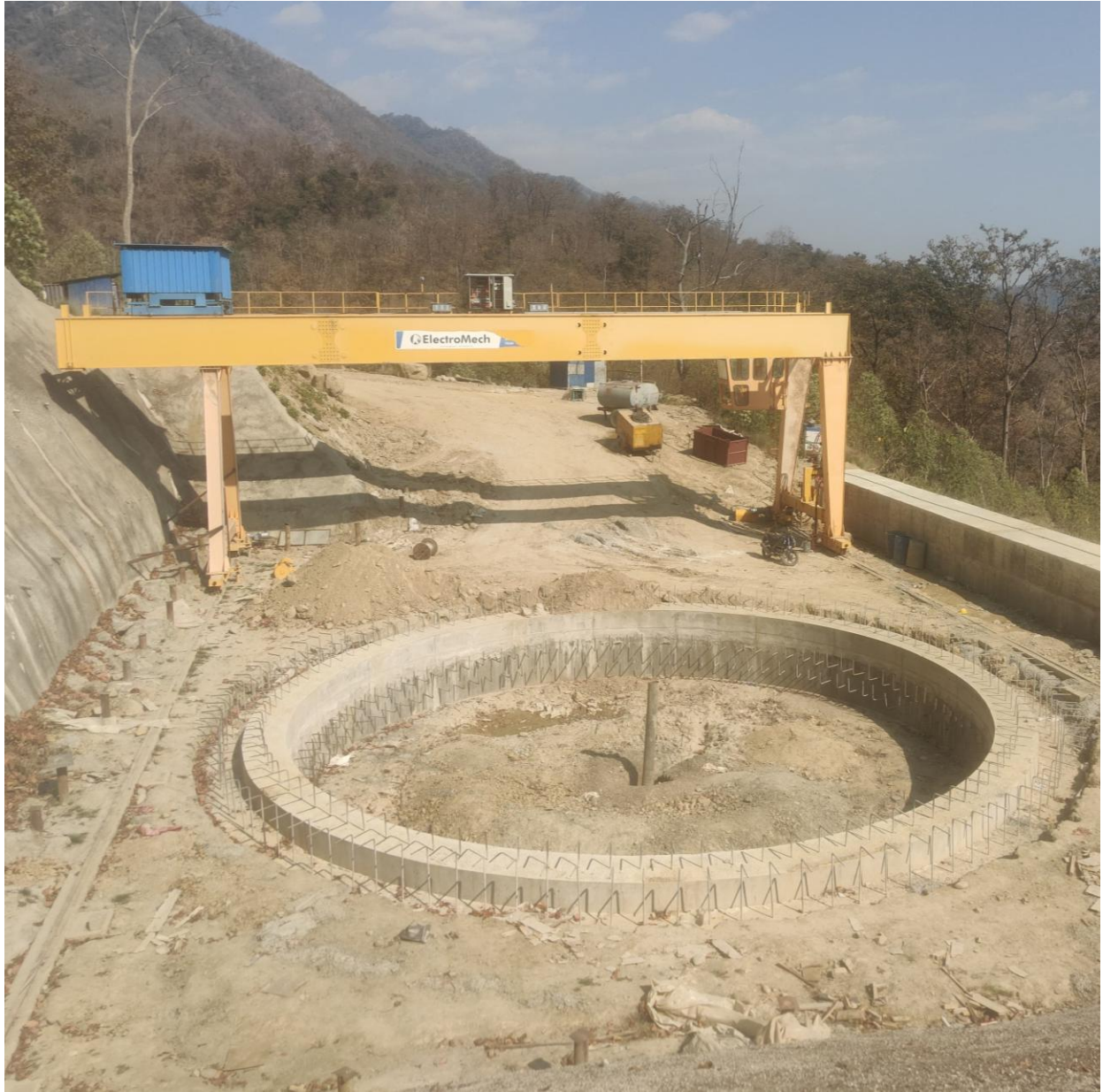
Figure 10 Gantry Crane installation at Surge Shaft
