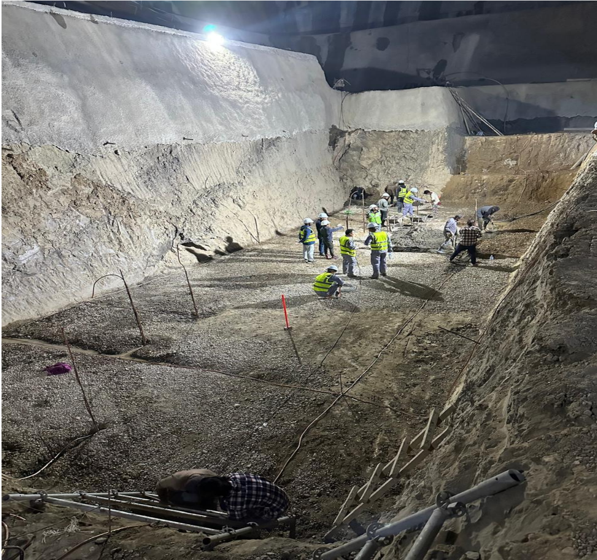
Figure 11 Grounding Installation works
