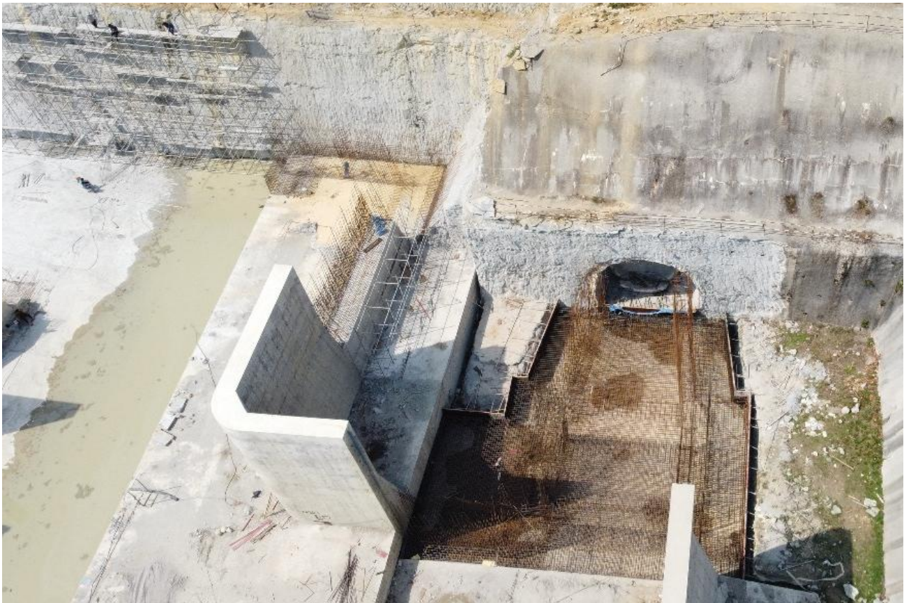
Figure 6 Forebay at Inlet Tunnel Portal
