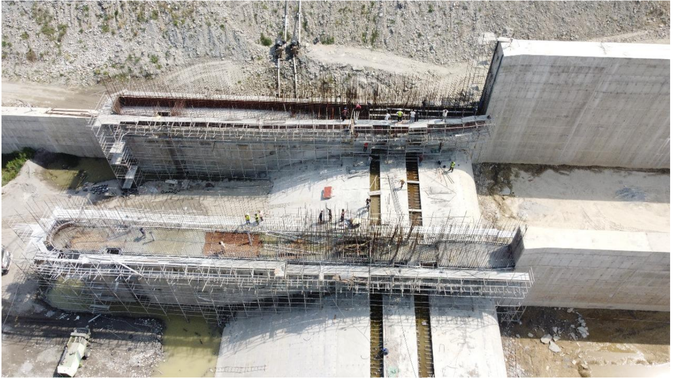
Figure 3 Spillway Ogee
