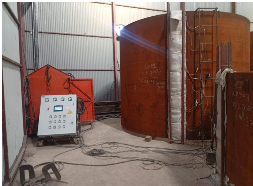
Figure 13 Penstock Pipe Rolling
