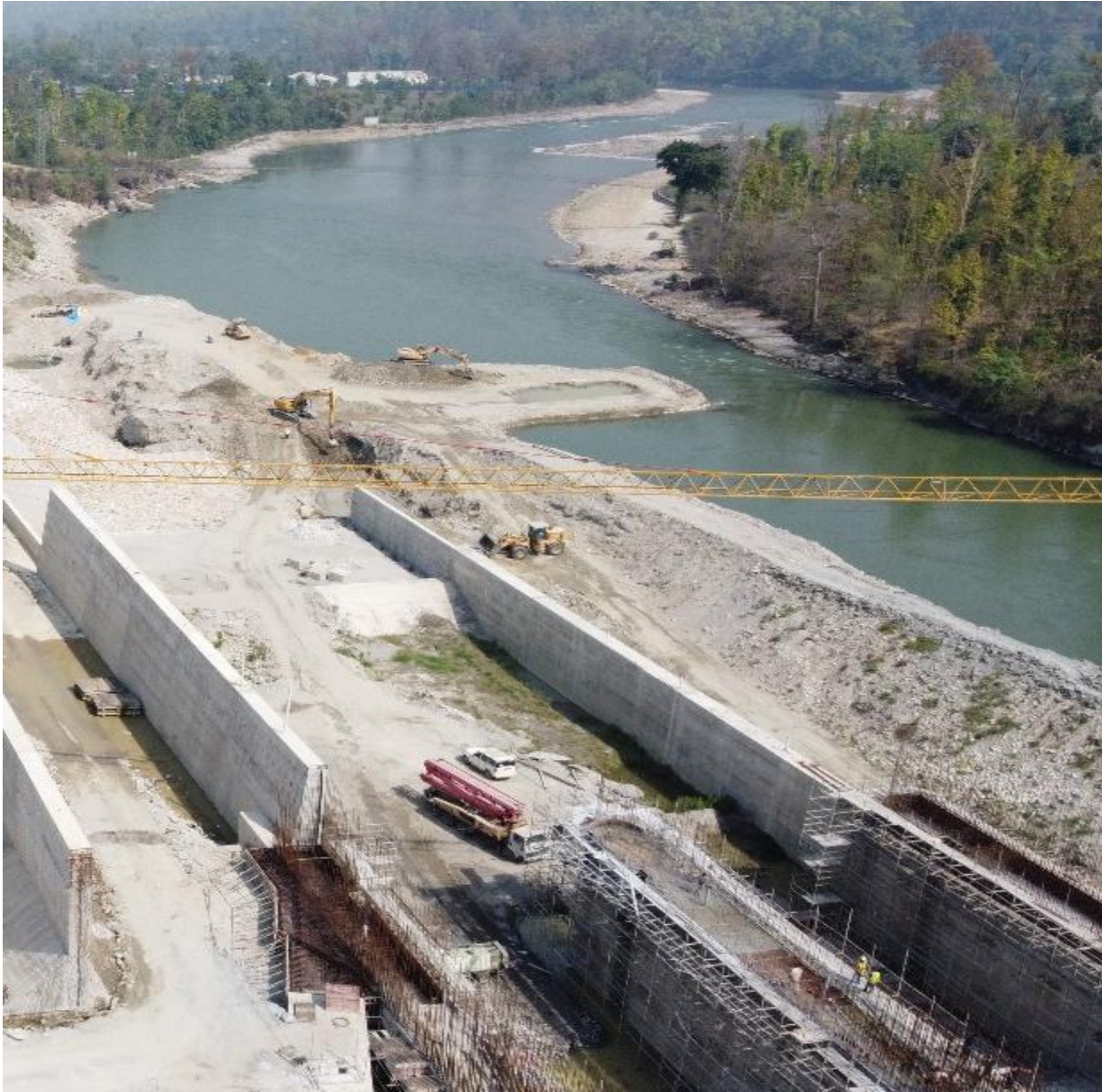
Fig 2: Headworks Cofferdam
