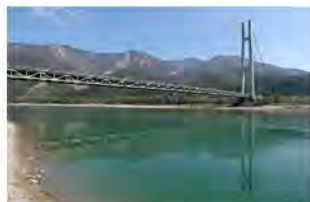
d. Two edges of the bridge
