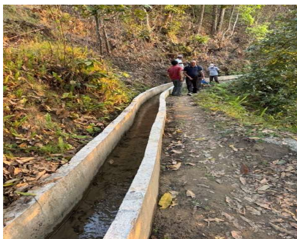
Figure 5: One of the sections supported by the Project for lining of canal.
