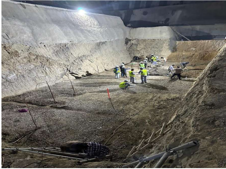
Grounding Installation Works
