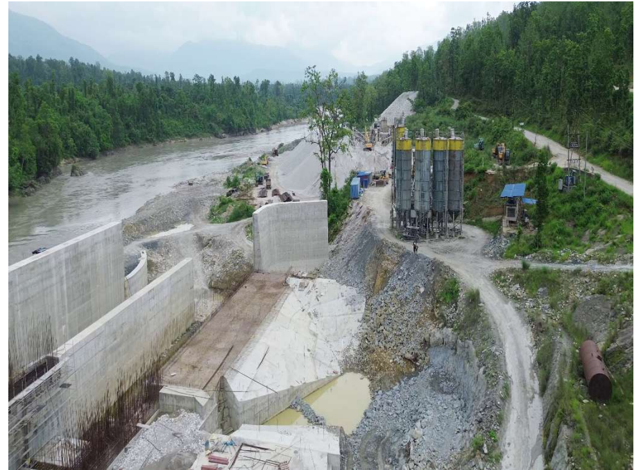
Headworks- Gravel Trap and Intake
