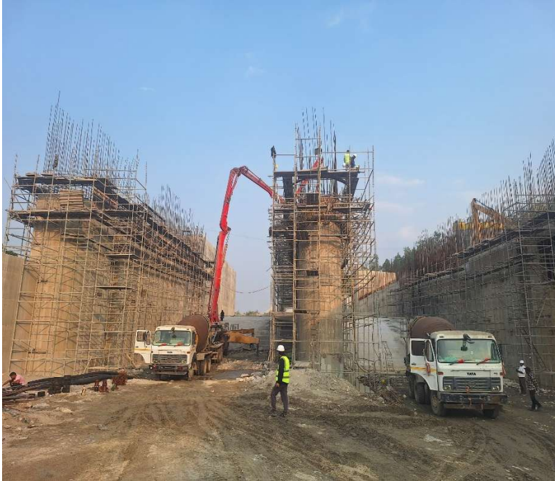
Headworks – Pier Construction
