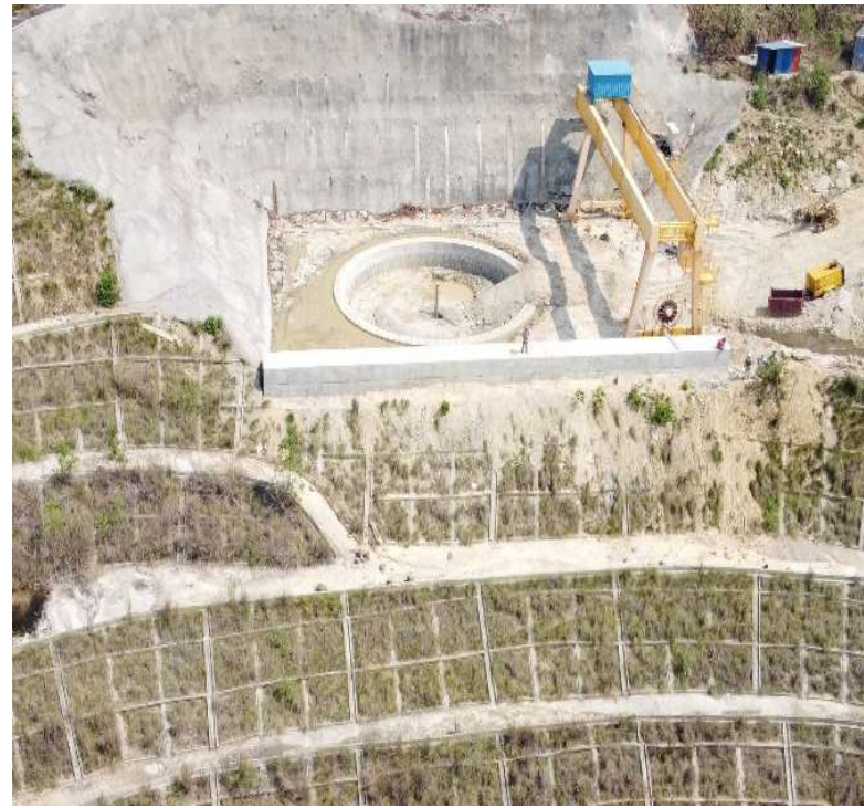
Powerhouse- Surge Shaft
