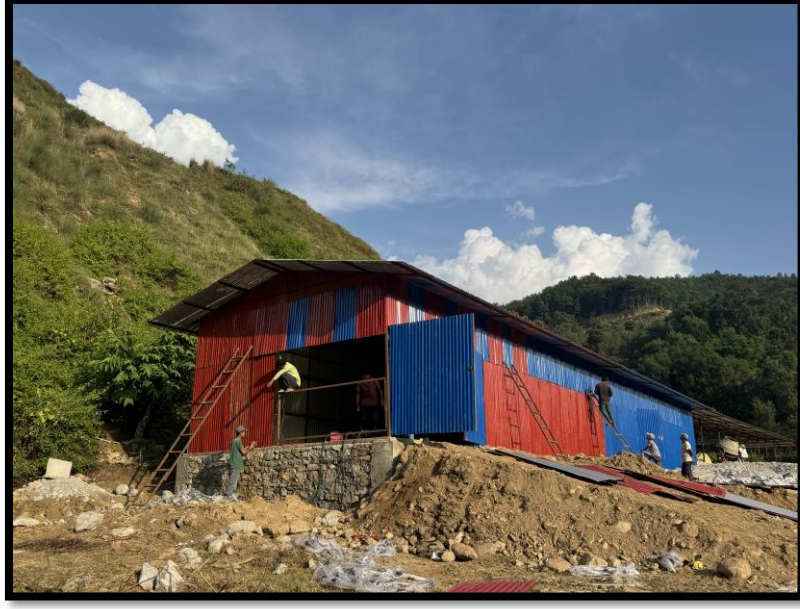
Completion of Storage House at Powerhouse Area
