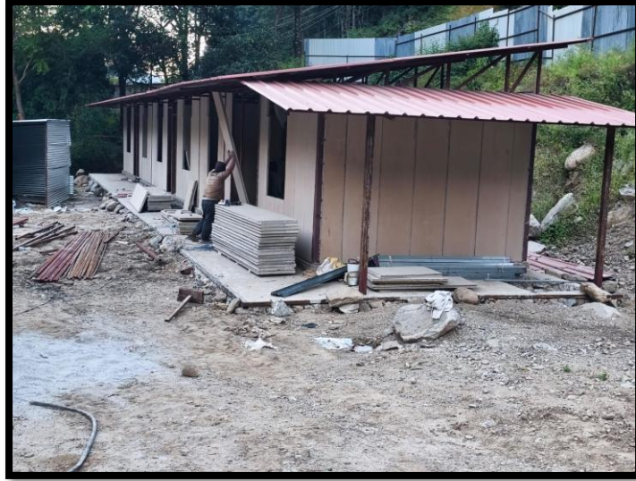
Cement Board Installation at Engineers Camp
