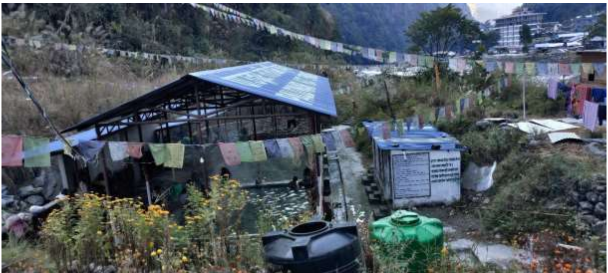
Photograph 1.1: Pond constructed and the area around Paudwar Tatopani, Myagdi
