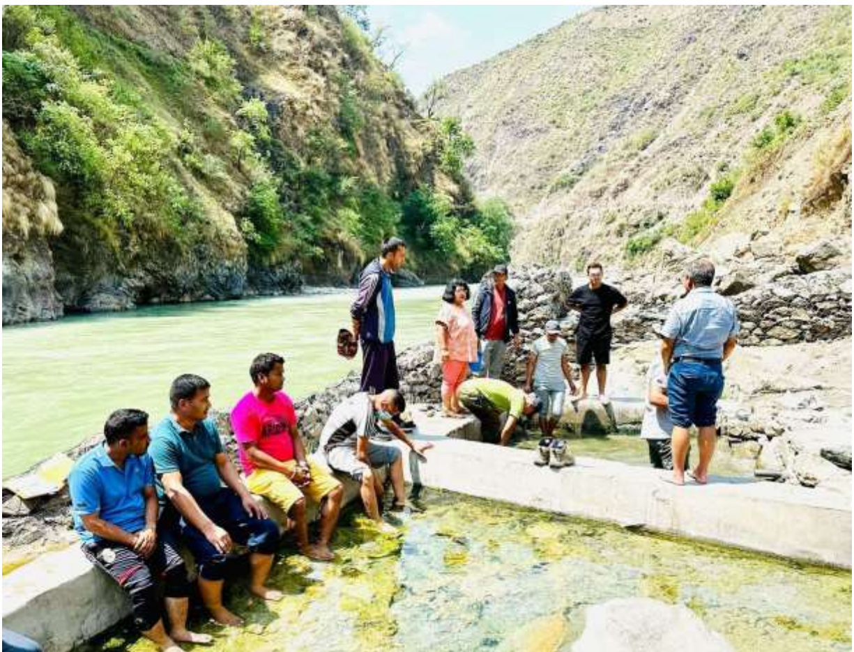
Photograph 1.1: Current situation of hot water spring source
