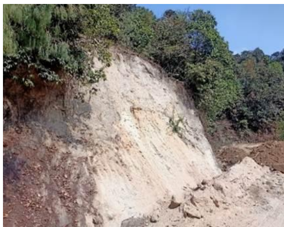
Figure 3- 4: Weathered augen gneiss bedrock exposed near to Mulkharka
