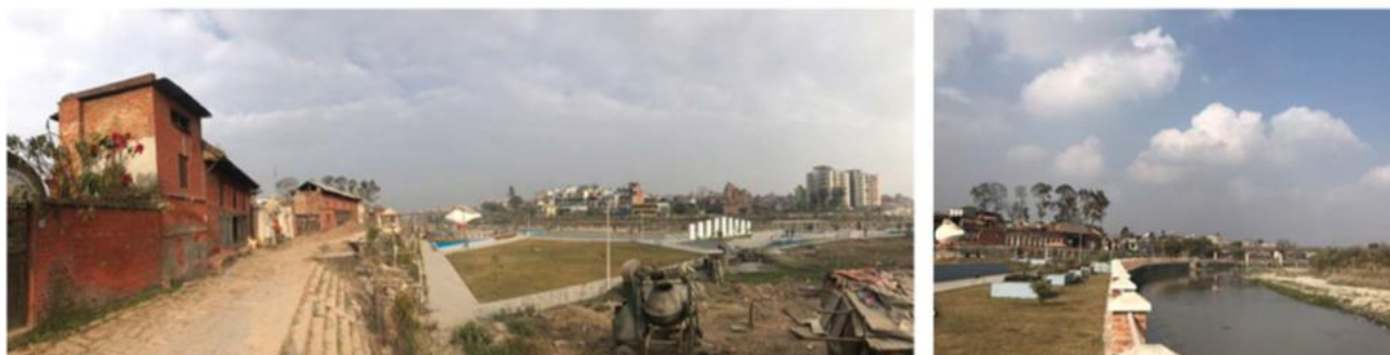
Figure 3- 19: Left: Shankha Park constructed on the reclaimed land, also seen are stone steps and bhakaro with few old house along the edge: Right: The width of the river is controlled using vertical walls and seen are the parapet walls along the Sankha Park
