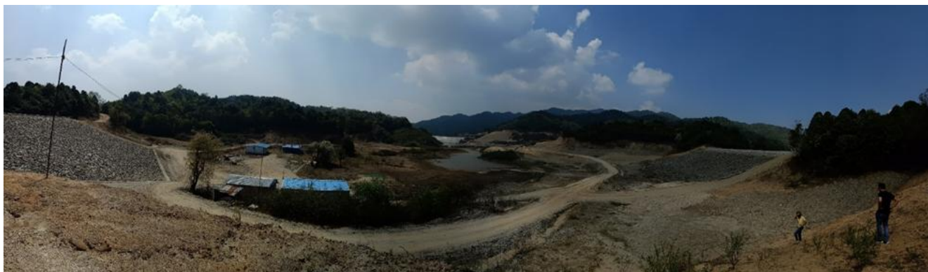
Figure 3- 20: Undergoing development of Dhap as a Recharge Lake near to Chisapani in Shivapuri National Park
