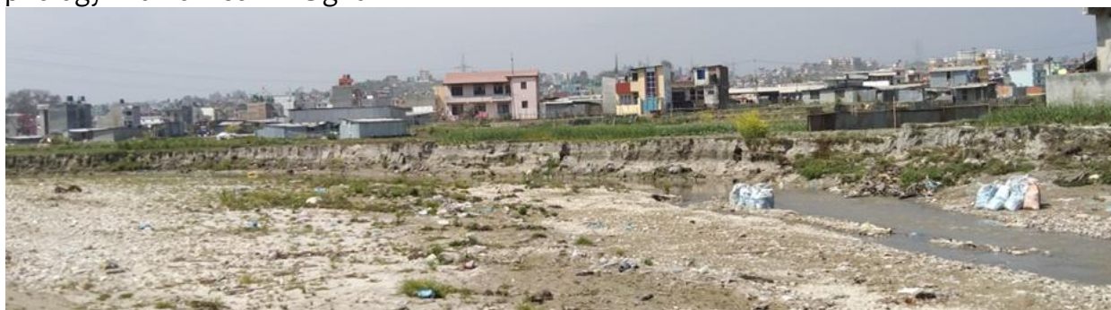
Figure 5- 10:River bank cutting by Manohara River
