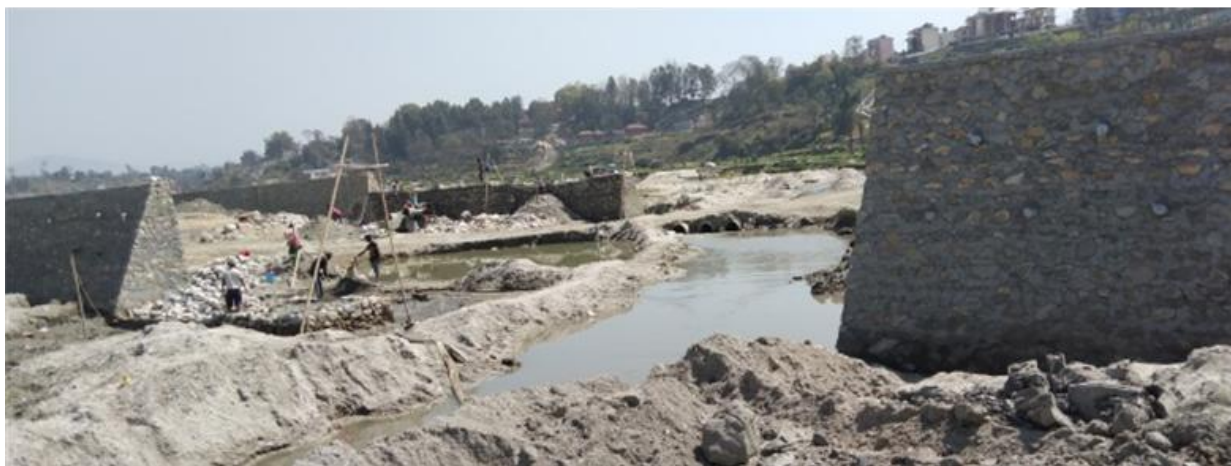
Figure 3- 17:River training works in Manohara
