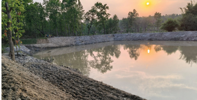
Water recharge pond under construction in Mainajor, Katari-5
