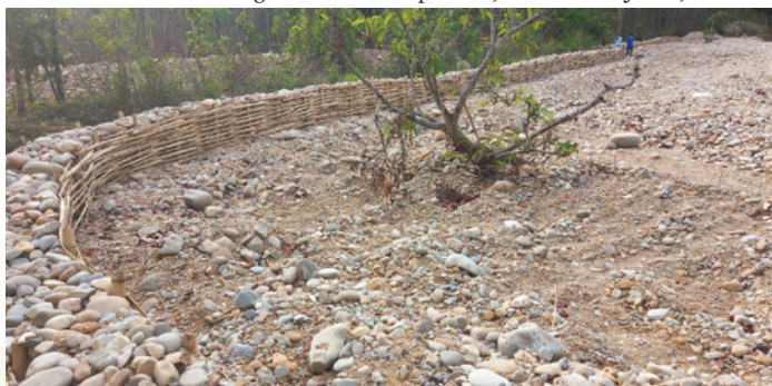
River Embankment using bamboo in Jutepani CF, Ratu River System, Bardibas
