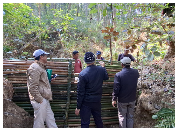
Checkdam using bamboo as part of the CERP interventions
