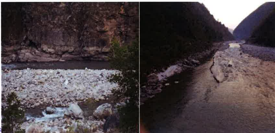
Photo 4-7: Pool habitat below dam site
