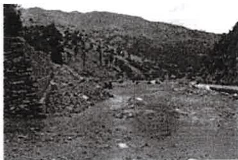
Figure 2-9: Construction Camp at Powerhouse site
