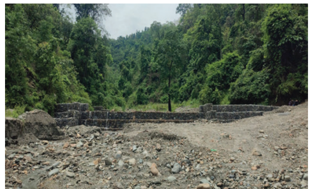
Pic 4: Check dam at Rong, Illam
