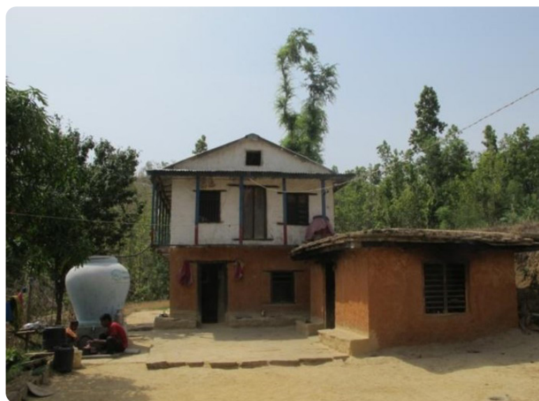
Figure 15: Rainwater harvesting in Ferrocement Tank and use
