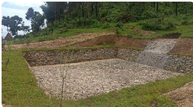
Figure 18: Water recharge pond
