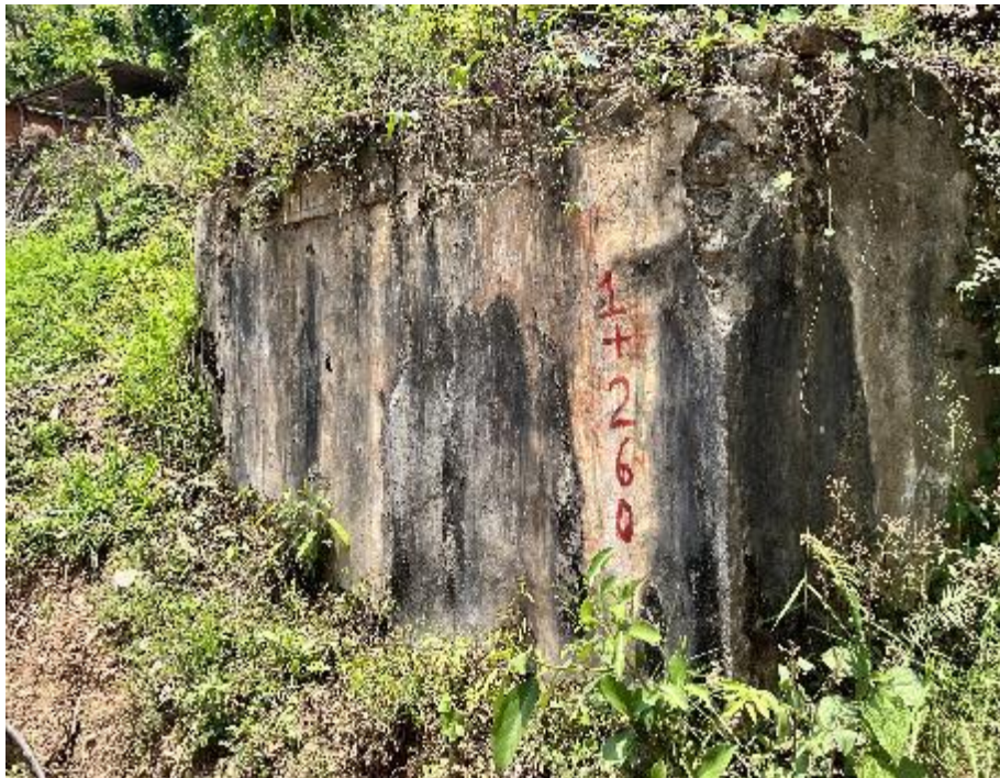
The existing water storage tank needs demolished
