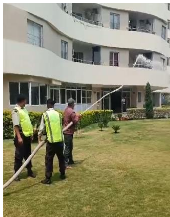
Testing of Fire Hydrant System
