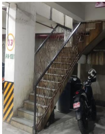
Evacuation staircase open to basement
