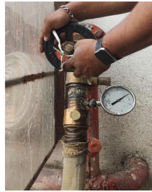
Flow testing of Fire hydrant with pressure gauge
