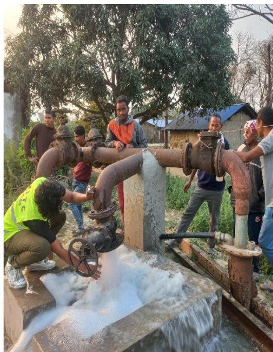
Deep Tube Well (New) - 100 m Depth, Jhapti
