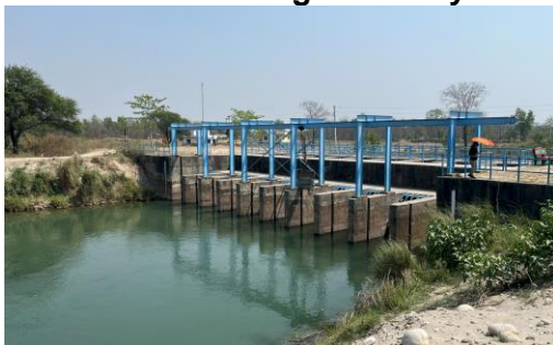
Intake gate before water enter structure
