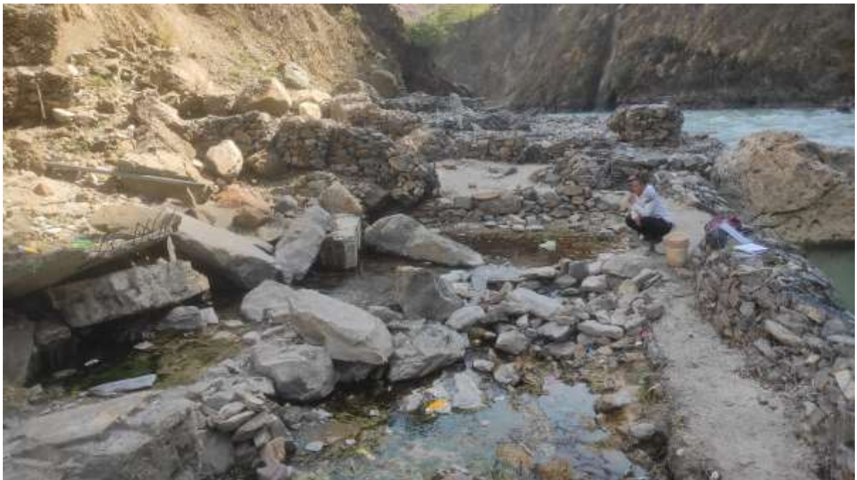
Photograph 5.70: The pond constructed at the Sunikot Totopani
