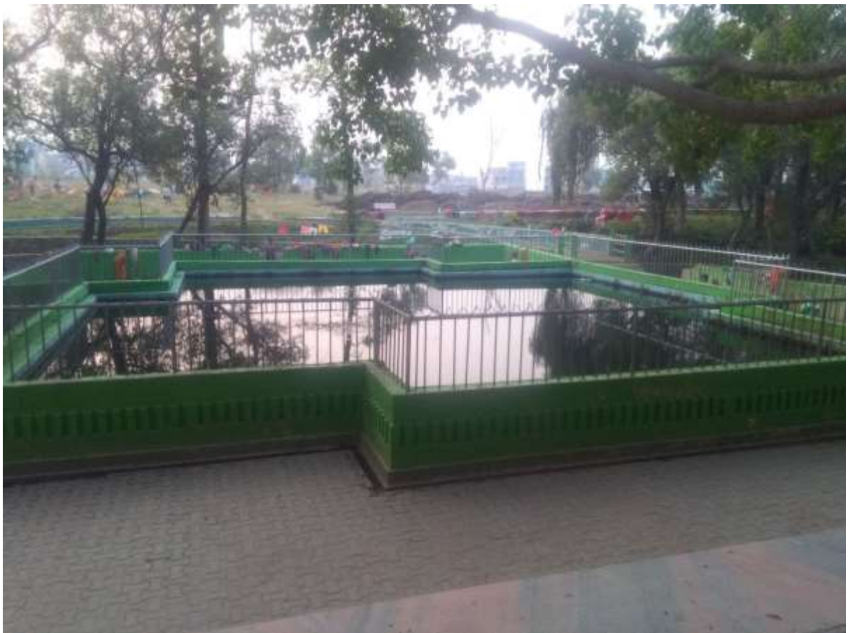
Photograph 5.64: Pond constructed at the Bulbule Taal
