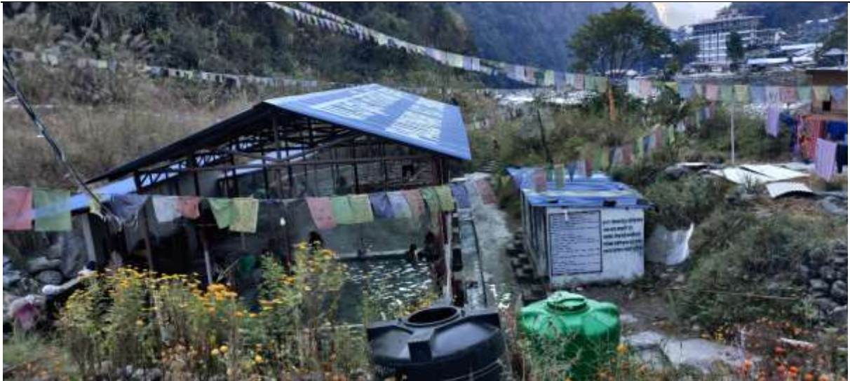
Photograph 5.22: Pond constructed and the area around Paudwaar Tatopani
