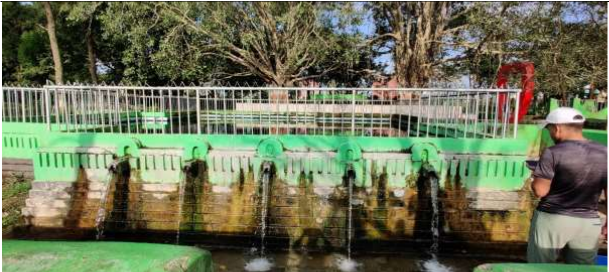
Photograph 5.63: Taps constructed at the Bulbule Taal
