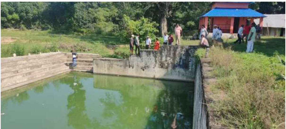
Photograph 5.47: Another view of the pond at the Tapta Kunda
