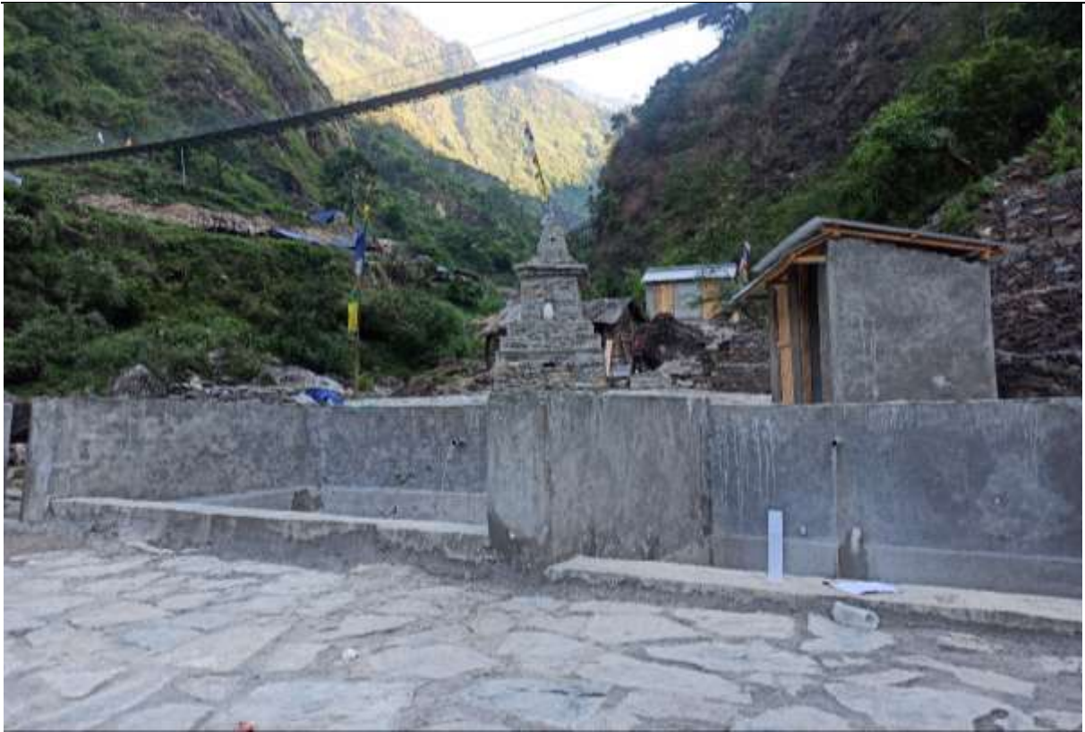
Photograph 5.5: Taps constructed at the Hindung tatopani
