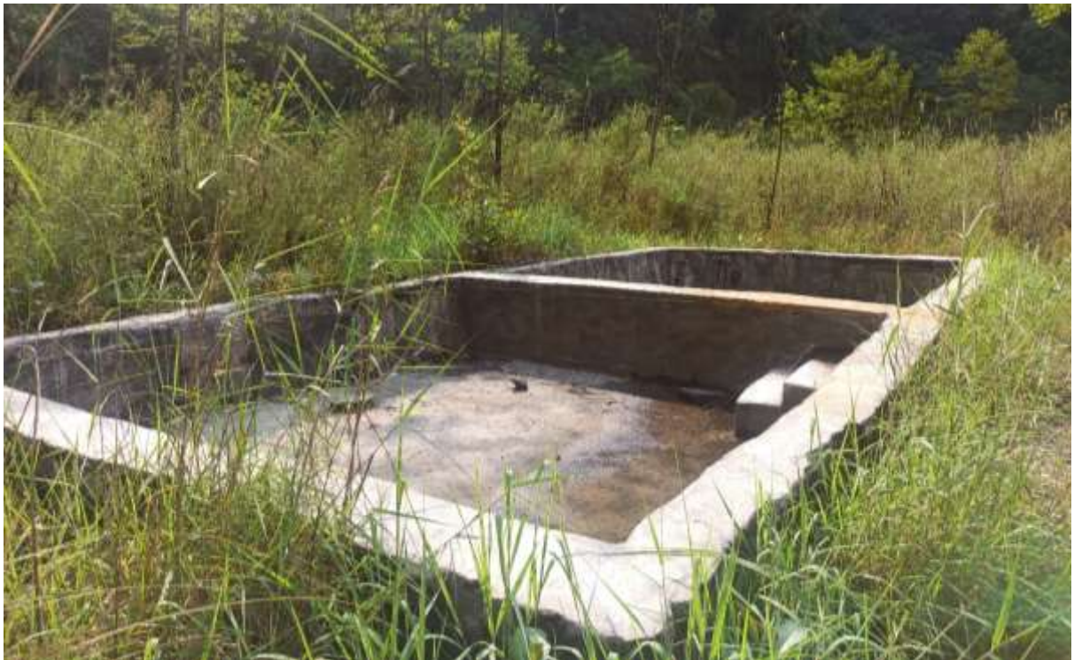
Photograph 5.18: Pond constructed for bathing purpose at Poje tatopani
