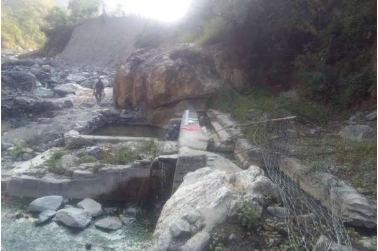
Photograph 5.36: Taps and pond constructed at the Jharna Tatopani
