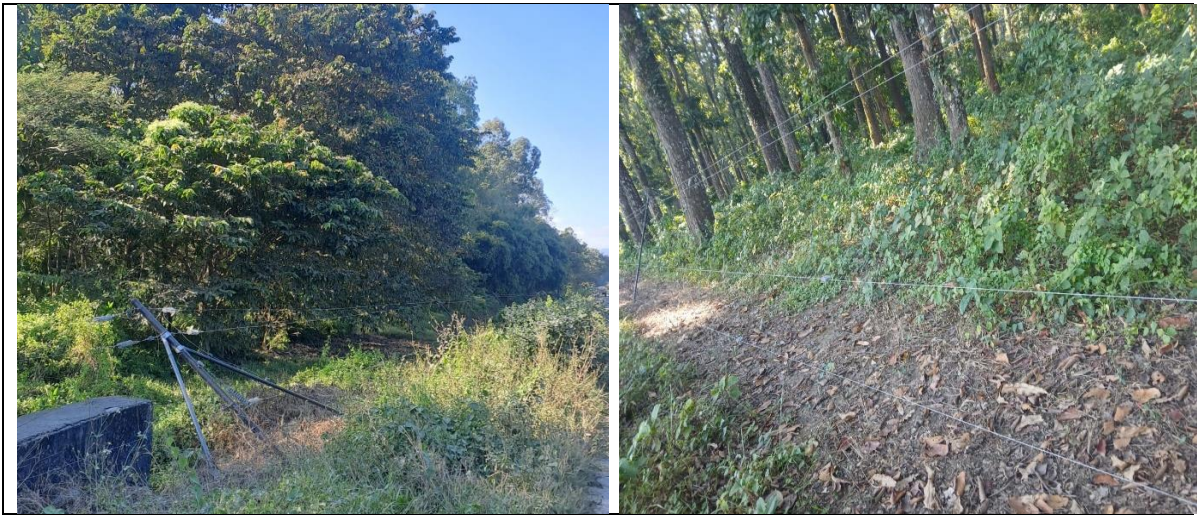
Figure 5-XIX: Fencing for wildlife along the Forest Edge of the Mechi Highway
