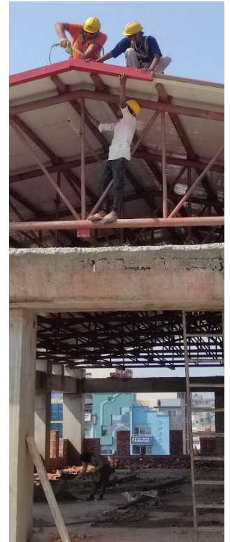
Working on roof, no proper safety gears
