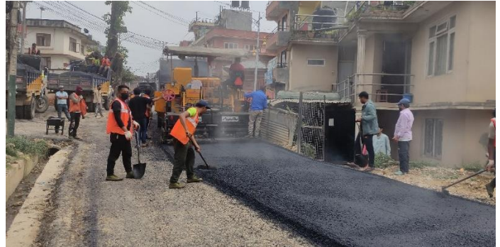
Spreading of bitumen
