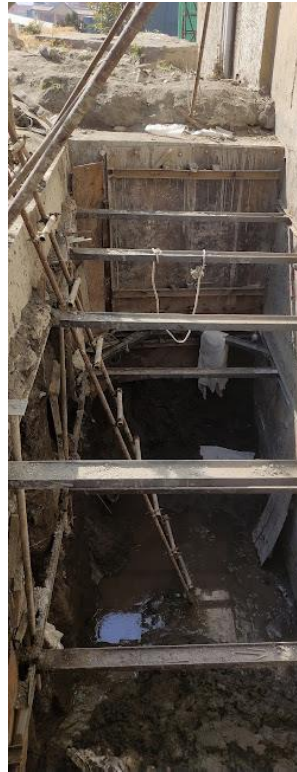
Excavated trench with protection work
