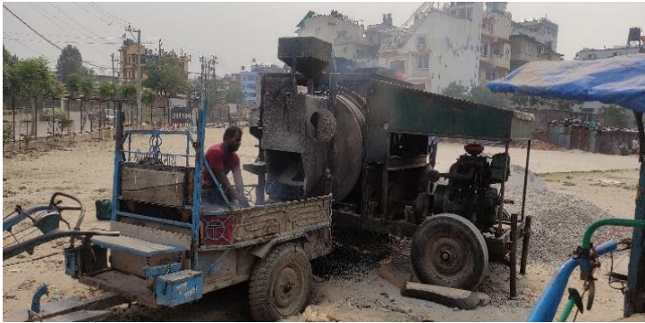
Production of asphalt concrete in urban road construction site, no PPE used by worker
