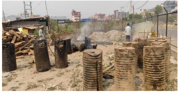
Traditional bitumen boiling work, no PPE used by workers
