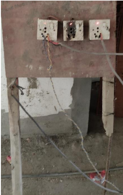
Unsafe electrical installations
