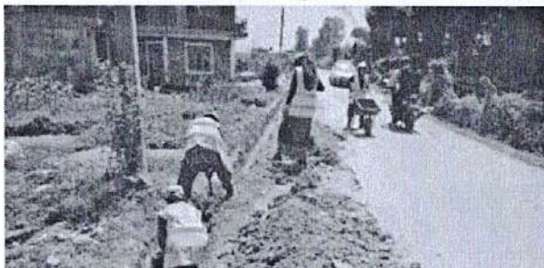
Clearing drainage ditches
