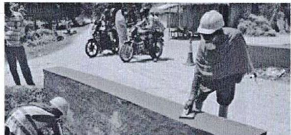
Clearing and repairing culvert
