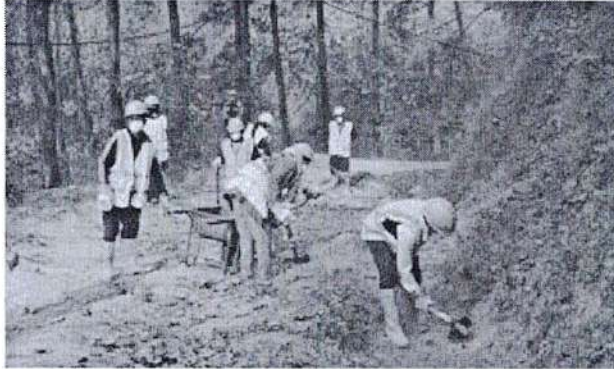
Construction of side drains
