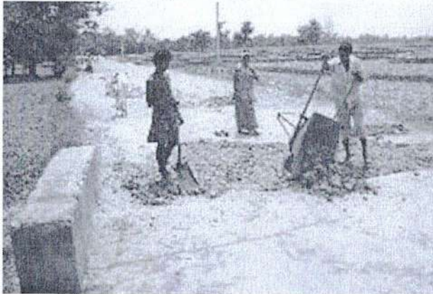
Repairing approach of culvert
