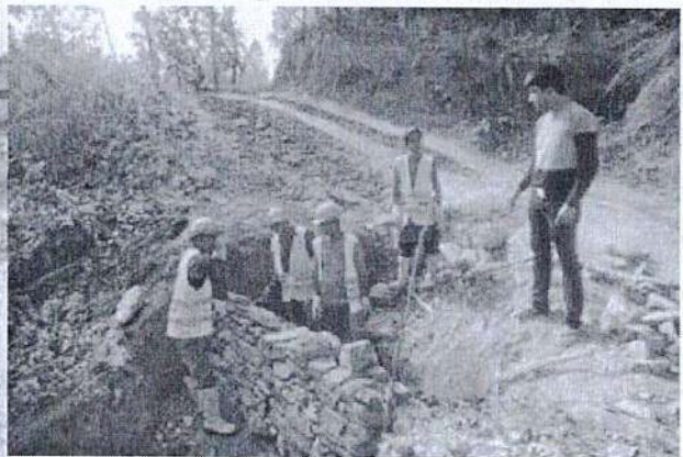
Minor protection work
