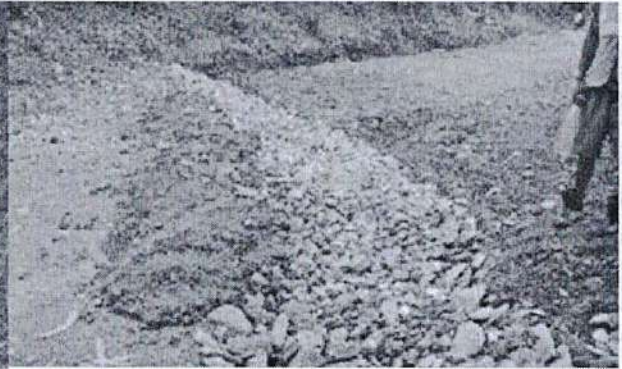
Construction of stone paved water crossings
