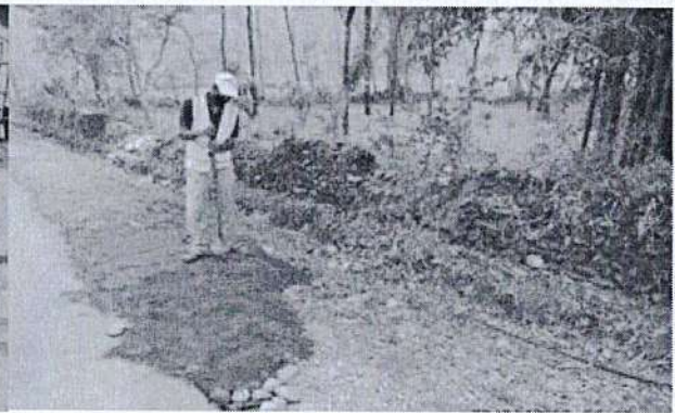
Repairing the road shoulder
