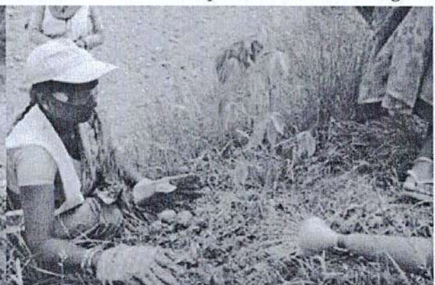
Protection of slopes by planting vegetation
