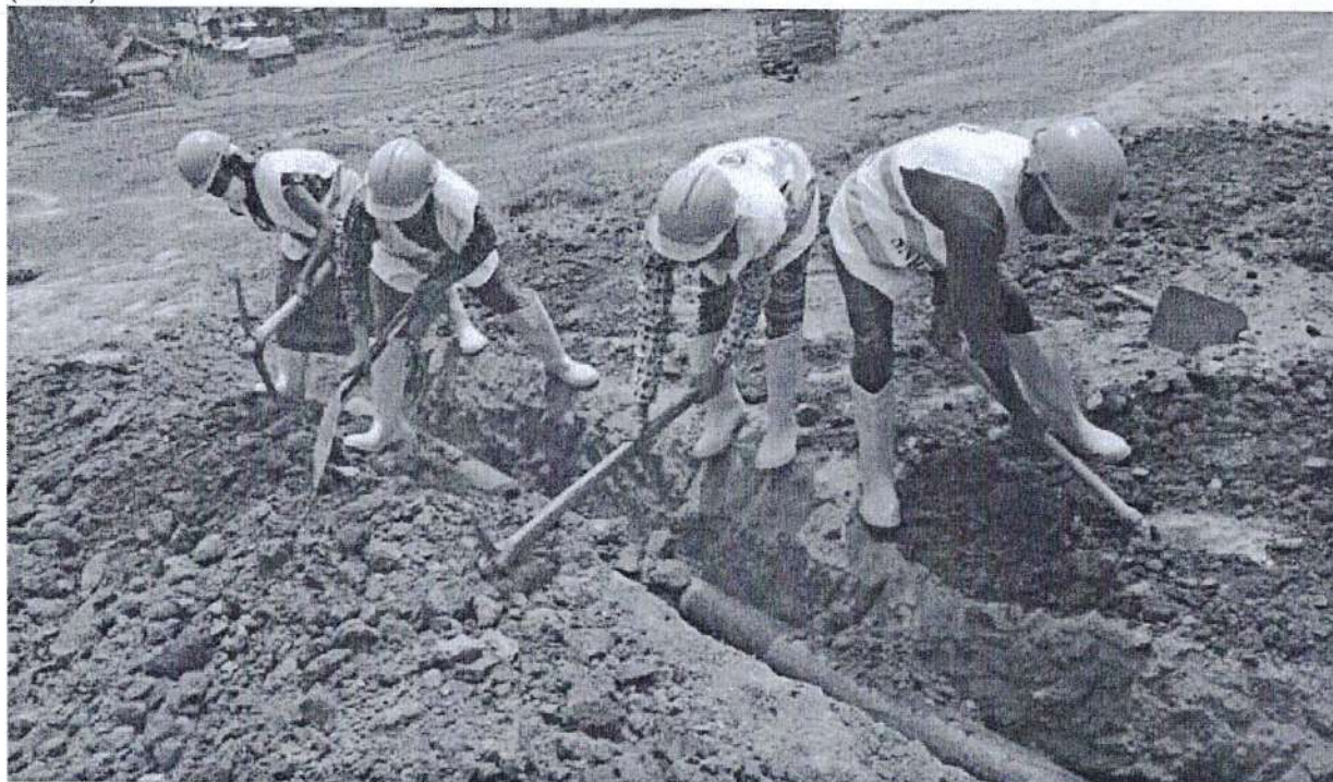
RMG members working for irrigation crossing
