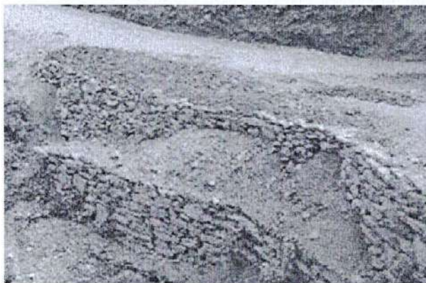
Construction of dry stone retaining walls
