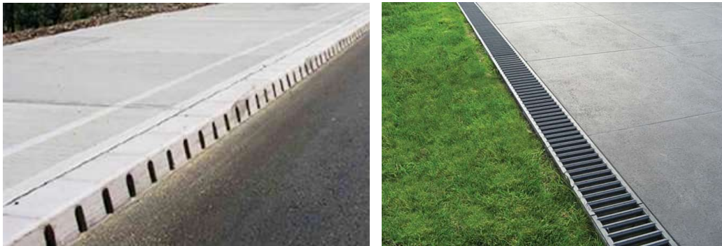
Figure 3-1 Slotted kerb drain and grated trench drain
