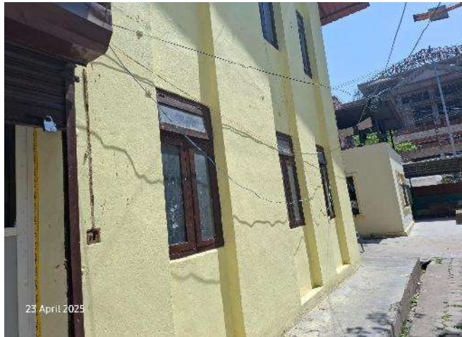
Trailing electrical cables across the building.
