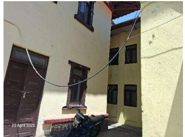
Trailing electrical cables across the building.
