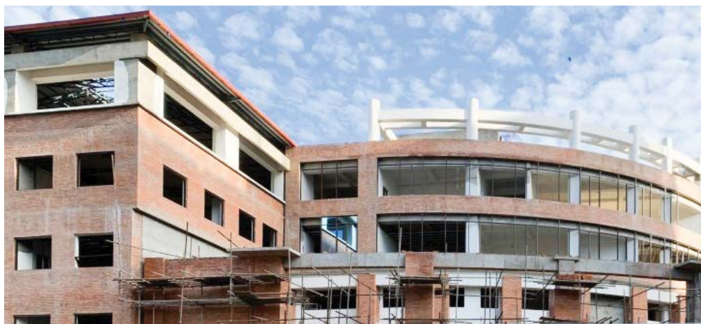
The multipurpose building under construction at Tripureshwar, Kathmandu
