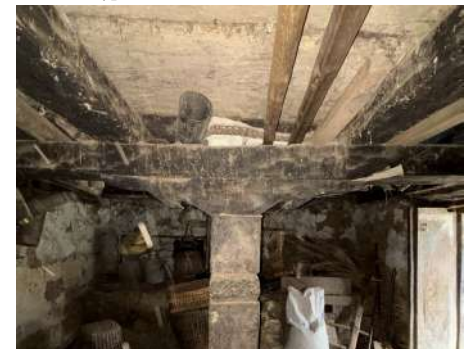
Typical Post and Beam Connection
