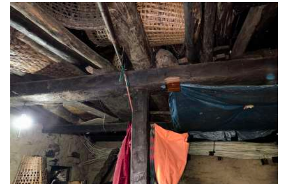
Typical Post and Beam Connection
