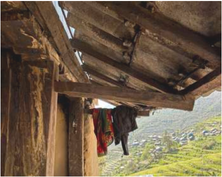
Timber Strut Supporting the Roof Projection
