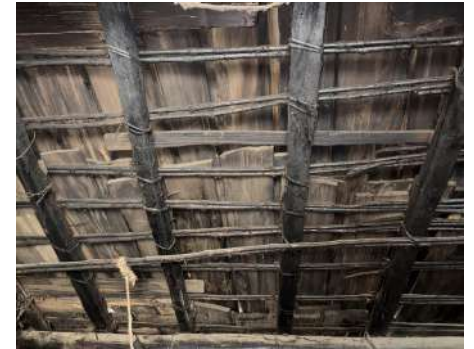
Panglep Roof Structure
