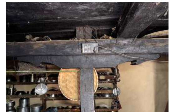
Typical Post and Beam Connection
