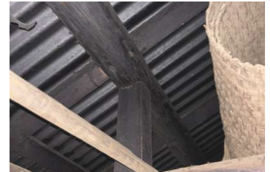
Typical Post and Beam Connection
