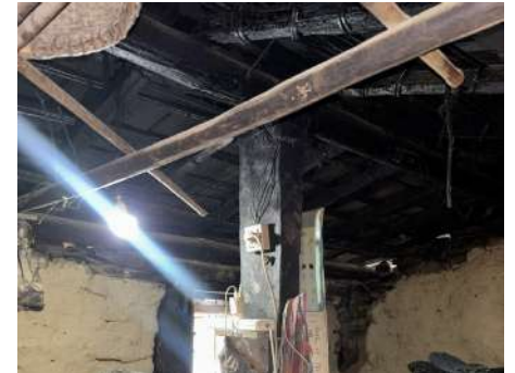
Typical Post and Beam Connection
