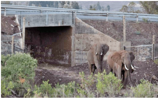
Figure2: Underpass in Kenya
