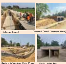
Syphon in Western Main Canal
