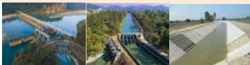
Weir Cum Bridge (315m)
