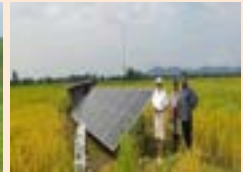
Photo 2: Diesel replaced after Solar PV pumping system
