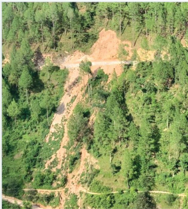
Landslide treatment with bioengineering techniques (After) – 2079/6
