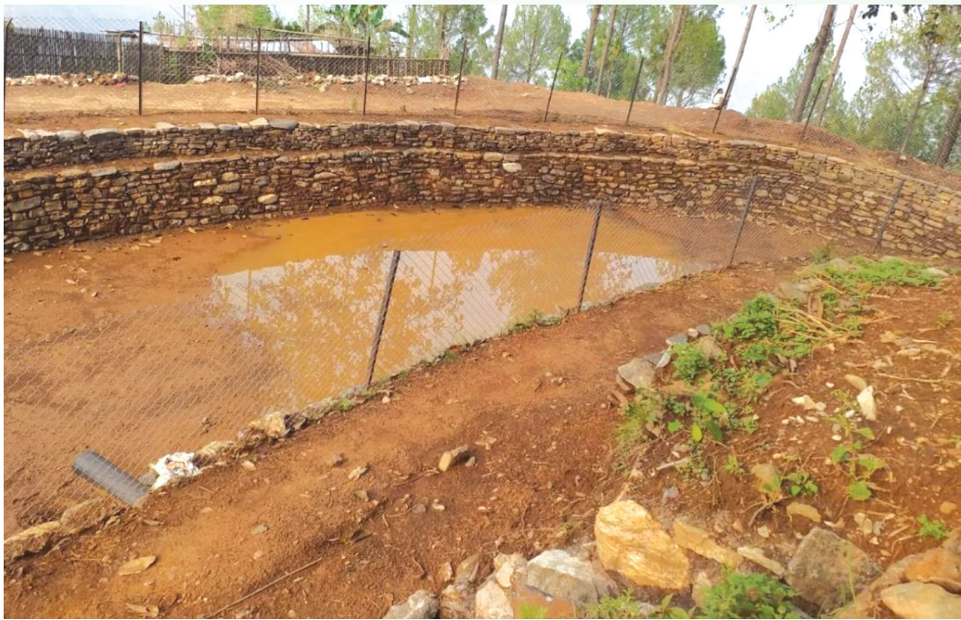
Construction of Water Recharge Pond at Chuliban, Dhankuta
