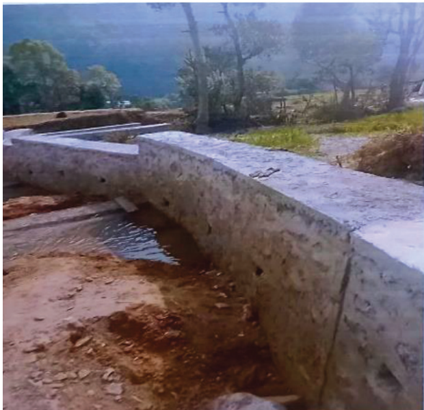
Constructed Stone Masonry RRM wall and Drainage Canal
