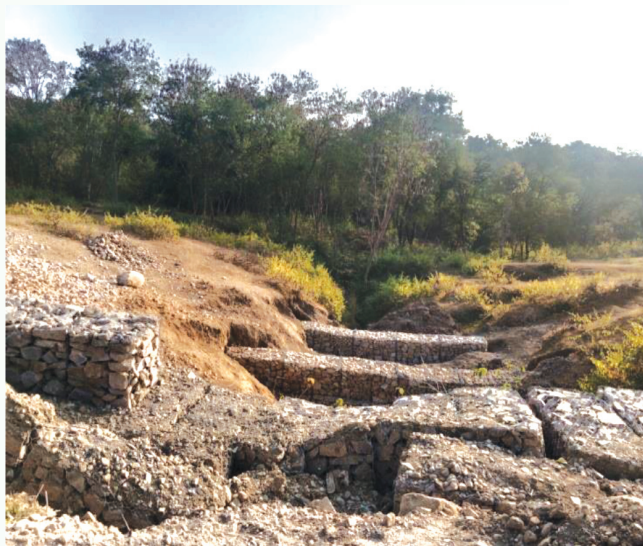
Damaged gabion retaining wall
