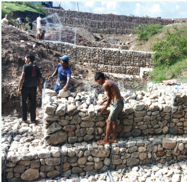
Repaired gabion retaining wall in Gully head and on-going gabion check-dam construction downstream
