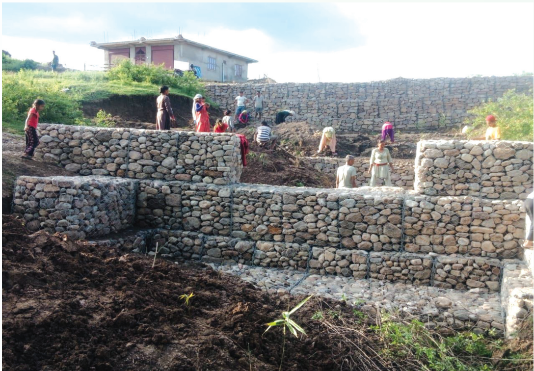
Completion of gabion retaining wall in Gully head and gabion check-dam construction downstream with bamboo clum-cutting plantation
