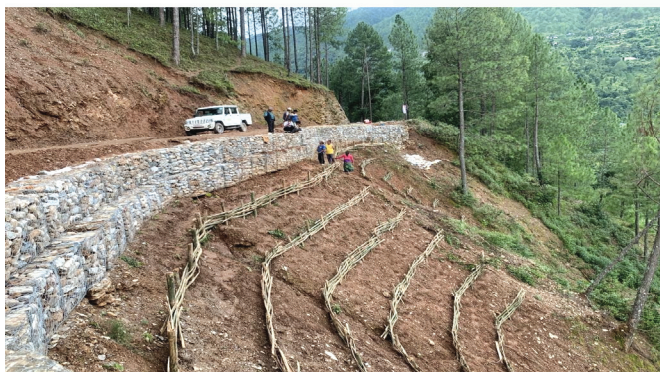
Retaining wall + Bamboo wattle fence (2079/4) - During Work
