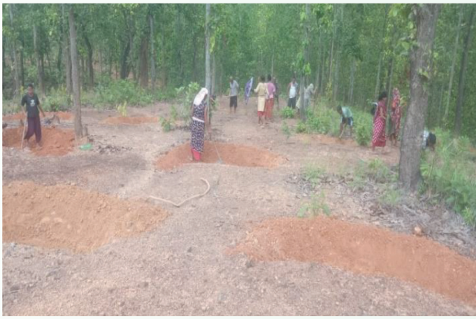
Participants digging eyebrow pit within forest land to retain moisture and prevent runoff and soil erosion
