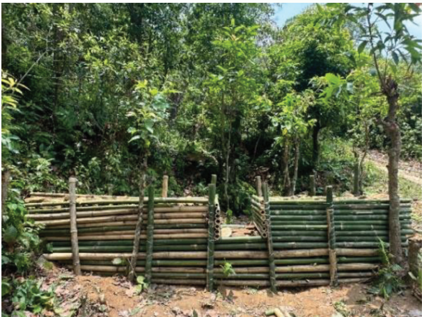
Participants prepare bamboo checkdam as low-cost soil conservation technique to control Gully erosion in Udayapur
