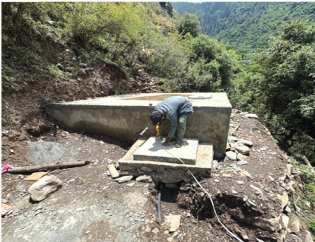
Construction of Intake, RVT, pipeline and Taps with protection of water source by gully control with local people's participation.
