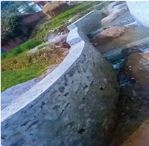
Constructed Stone Masonry RRM wall and Drainage Canal
