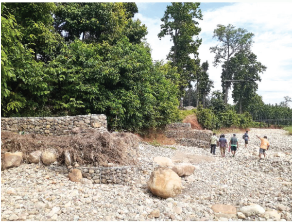
In F.Y. 2075/76, bamboo plantation and gabion embankment were carried out at Pattharkhola, Hupsekot-1, Jugepani, photo taken on: 2076/04/14 BS
