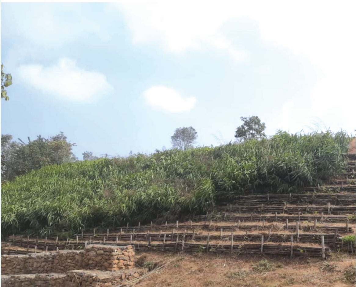
Bamboo crib wall and broom grass plantation
