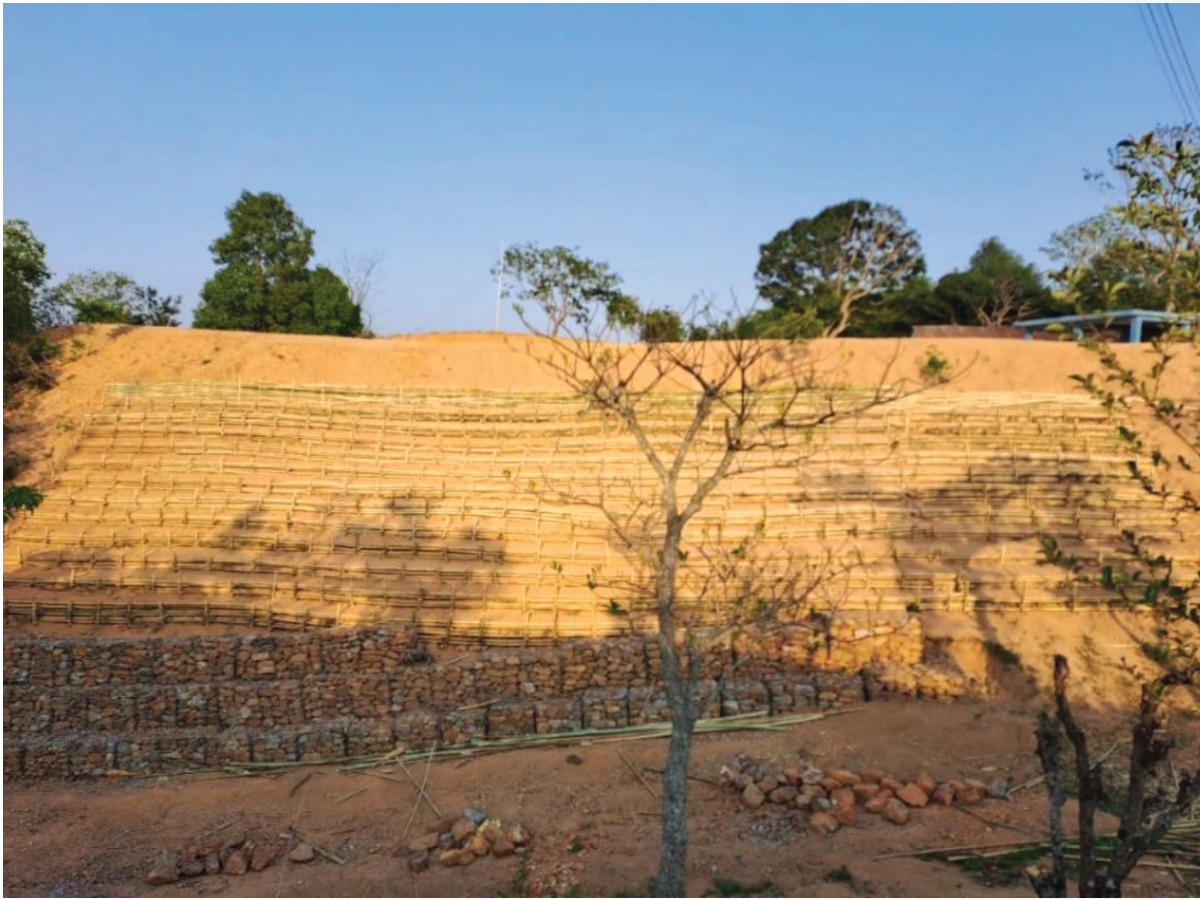
Site Preparation for Broom Grass Plantation on Bamboo crib wall
