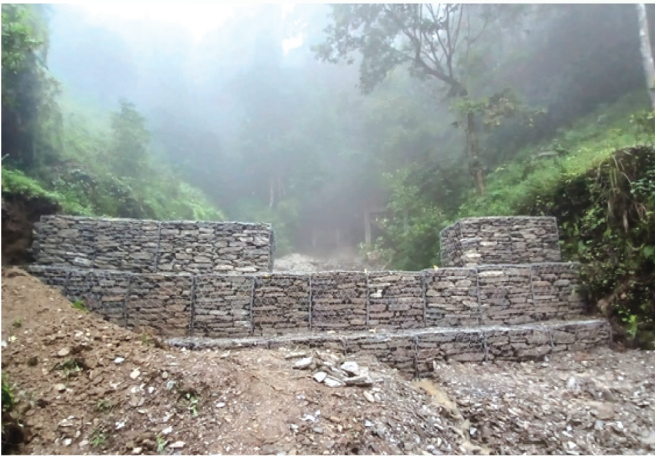
Landslide Treatment, Annapurna 4, Bhadaure, Kaski
