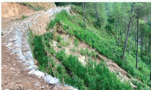
Retaining wall + Bamboo wattle fence (2079/6) - After Work
