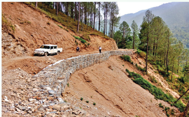
Gabion Retaining wall (2079/2)-During
