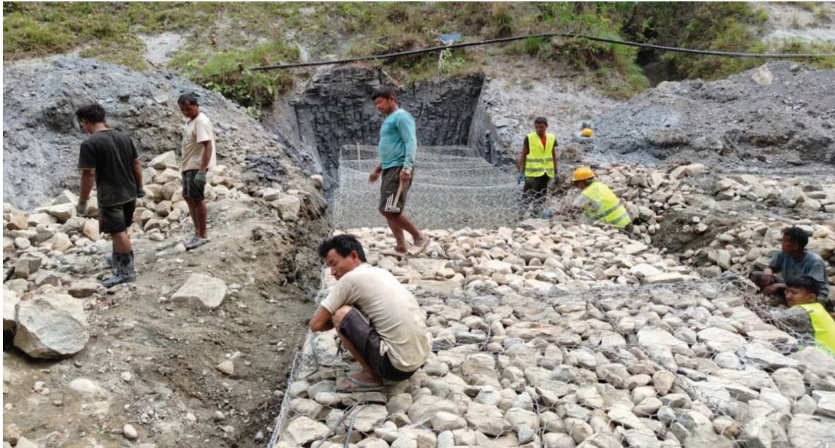
Runoff harvesting dam is currently under construction at the upstream terminus of the river embankment to intercept surface flow, reduce downstream sediment transport, and enhance groundwater recharge
