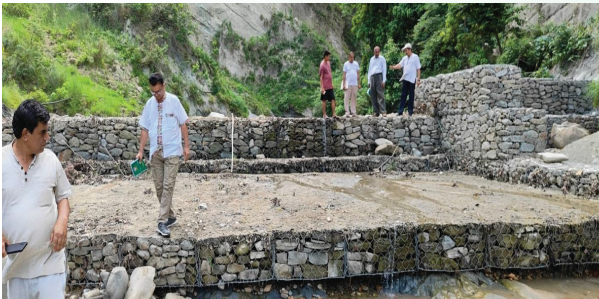
Within a three-month period, the runoff harvesting dam accumulated approximately 1,200 m 3 of sediment, effectively doubling the surface water retention upstream while reducing downstream sediment transport by nearly 50%.
