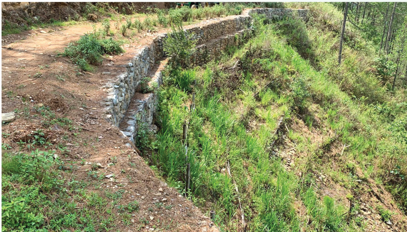
Retaining wall + Bamboo wattle fence (2082/3/1) - After Work
