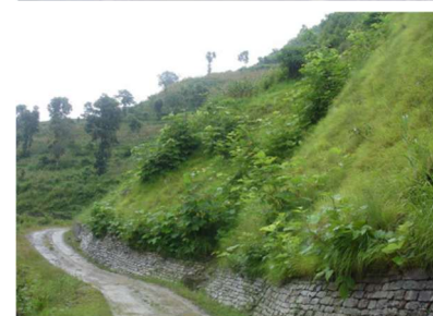
Fig: Slope after stabilization
