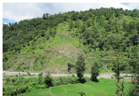
Slope Stabilization after Bioengineering
