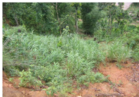
Slope stabilization after bioengineering
