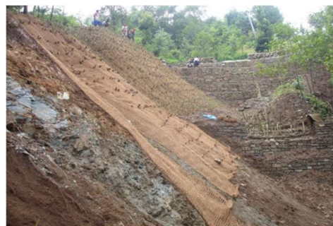
Gabion check dams, jute netting and grass plantation (Before and after)
