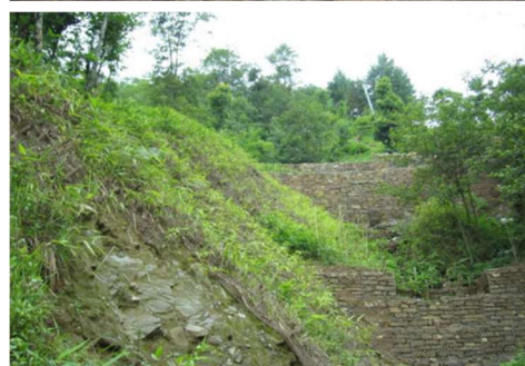
Live check dams, jute netting and grass and tree plantation (Before and after)
