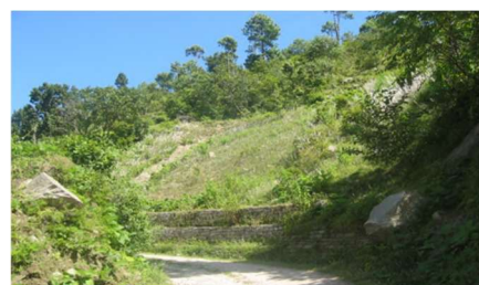
Before and after implementation of bioengineering
