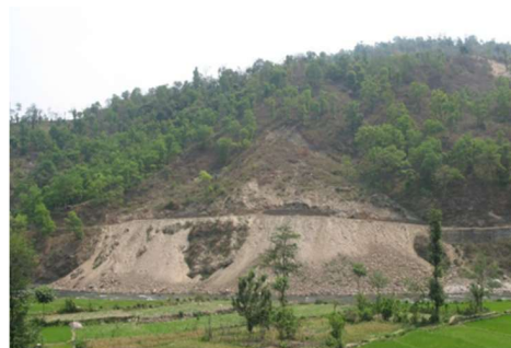
Slope before implementation of bioengineering
