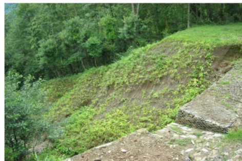
Gabion check dams, jute netting and grass plantation (Before and after)
