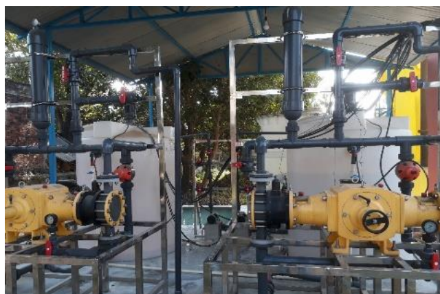
Chlorine Dosing System
