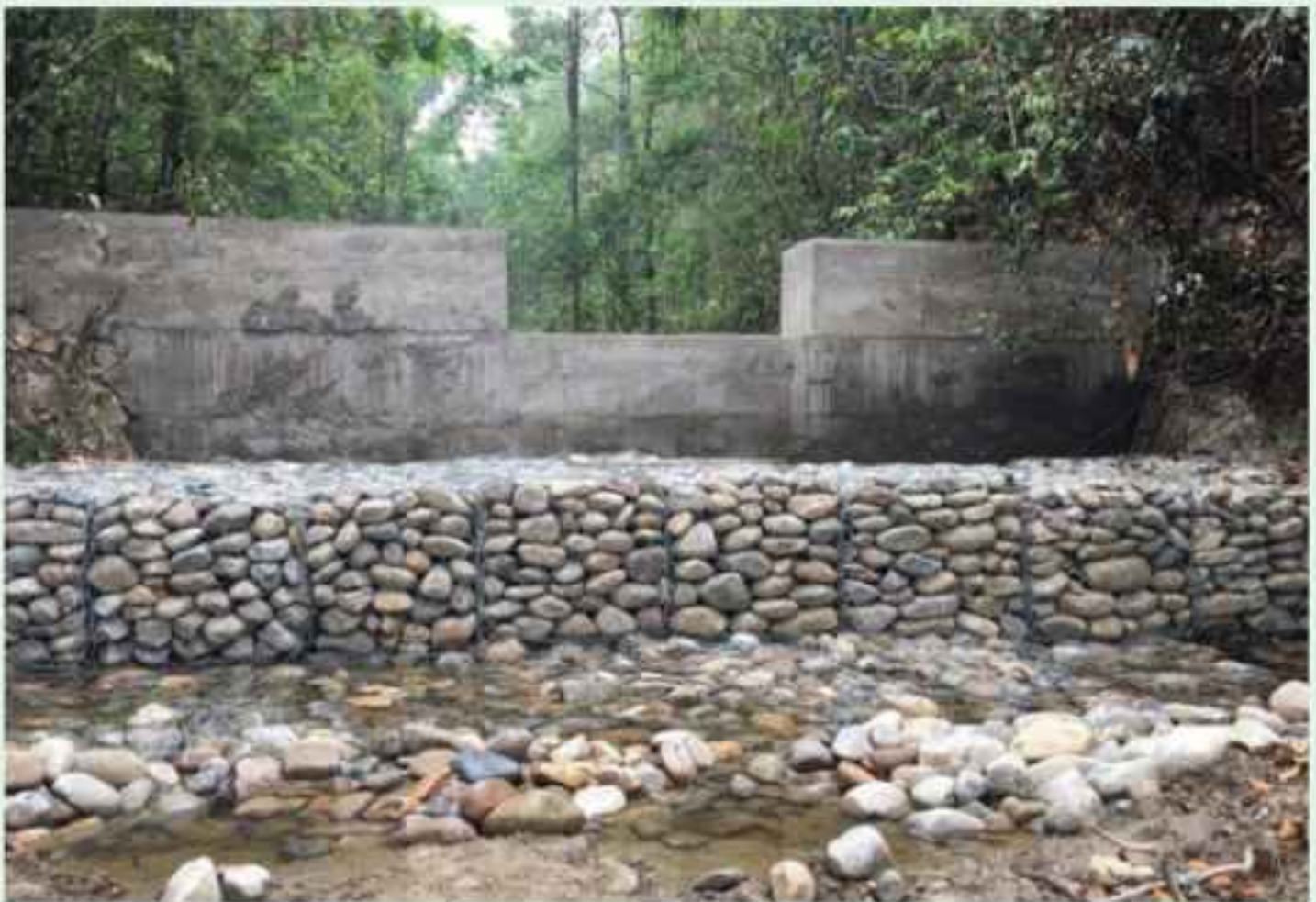
Run-off harvesting Dam, मरिण गा.पा., सिन्धुली
