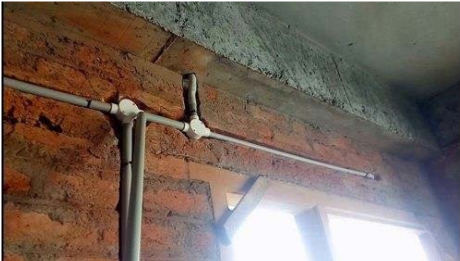
Figure 5.9: Concealed conduit wiring
