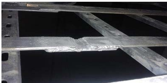
Figure 4.15: Strip earthing
