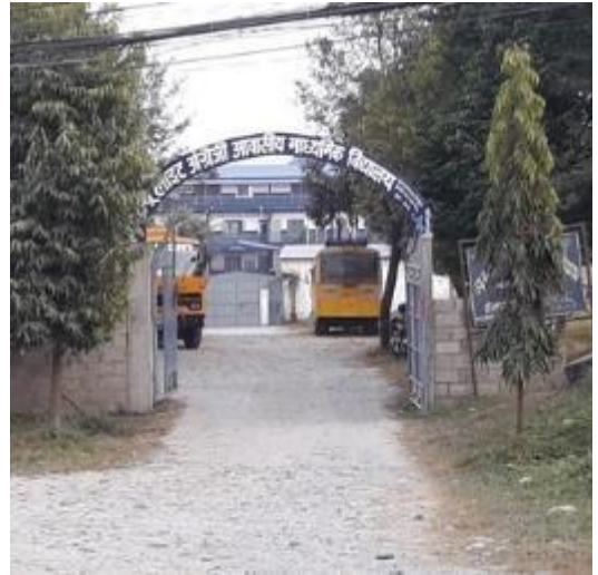
School in road alignment
