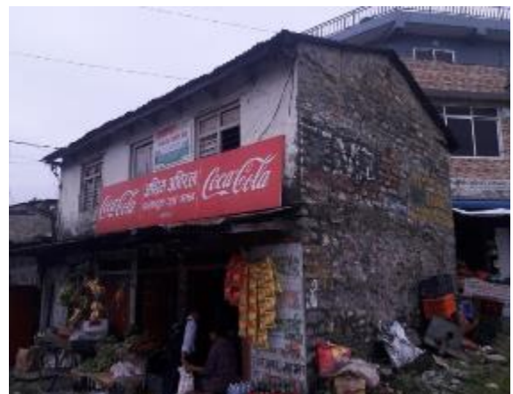
Road affected house at Sisuwachok
