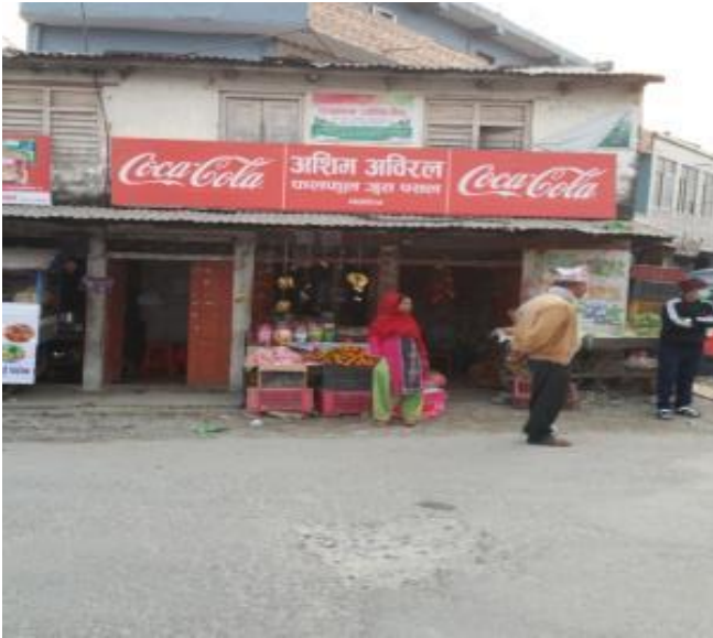
Affected house and shops, SisuwaChowk
