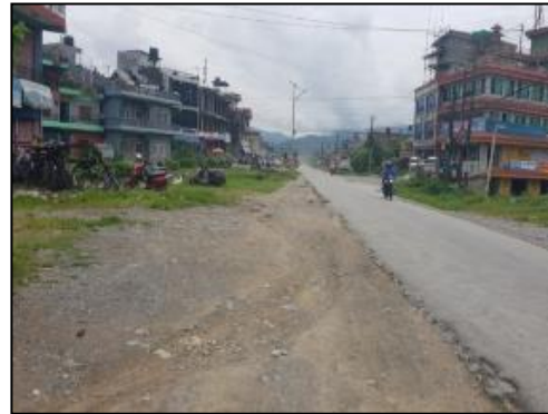
Road Near Sisuwa at 0+900
