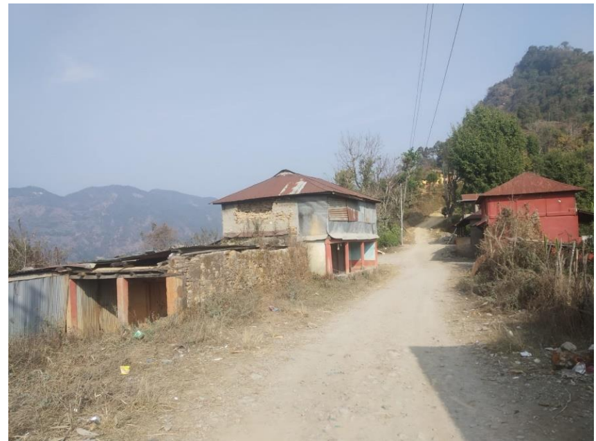
House falls within the RoW where the existing road width finalised to 4.5 m at Ch:5+790
