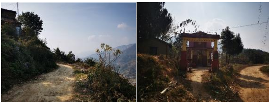
Existing road condition
