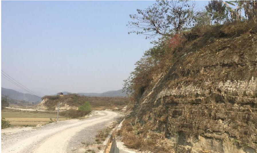
Pic 9: Landslide Prone Area, Kameromato, Ward no. 9,
