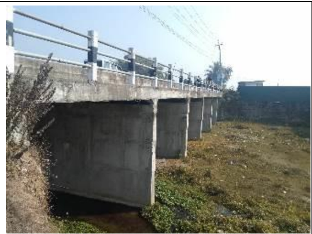
Photo 2: Existing bridge over Sehora khola
